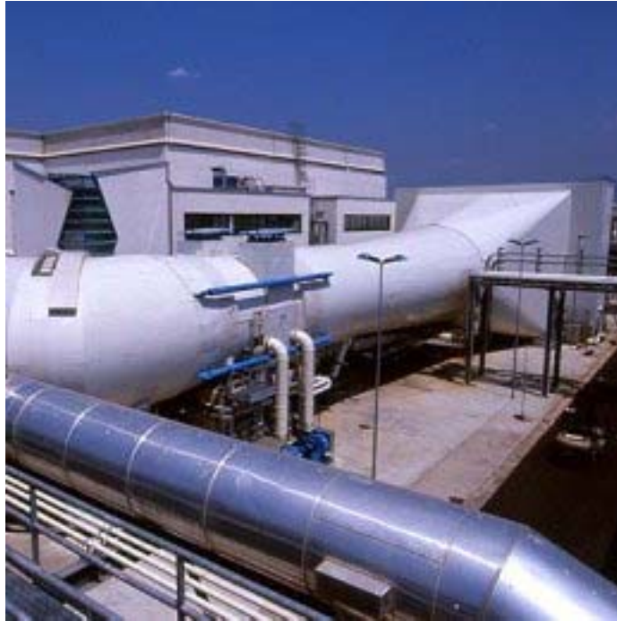
Icing Wind Tunnel (IWT), Italian Aerospace Research Center (CIRA), Capua, Italy.
