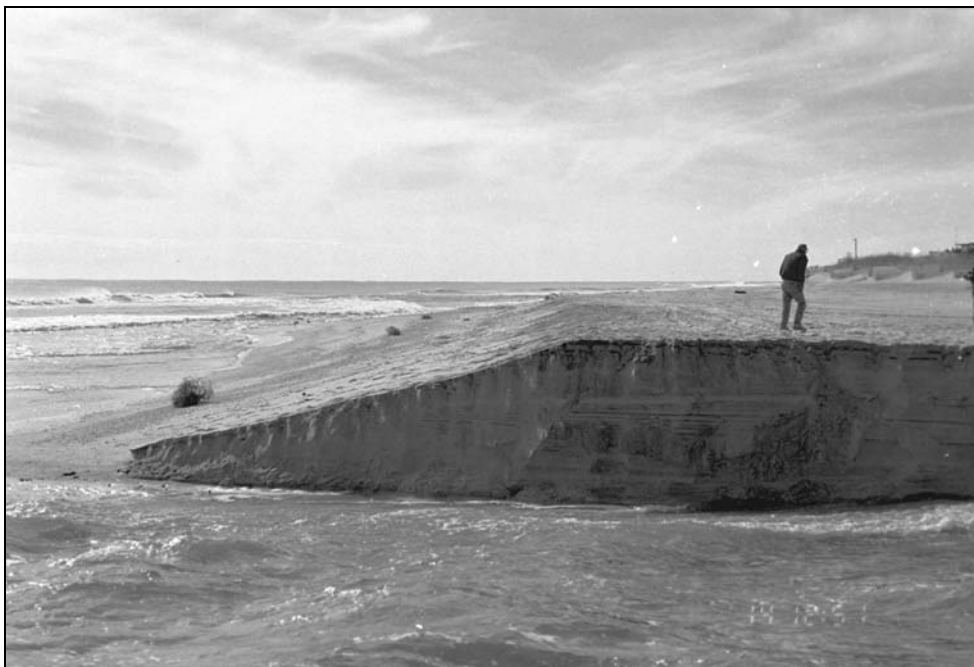
b. Looking east, at breach cut through the beach berm.
