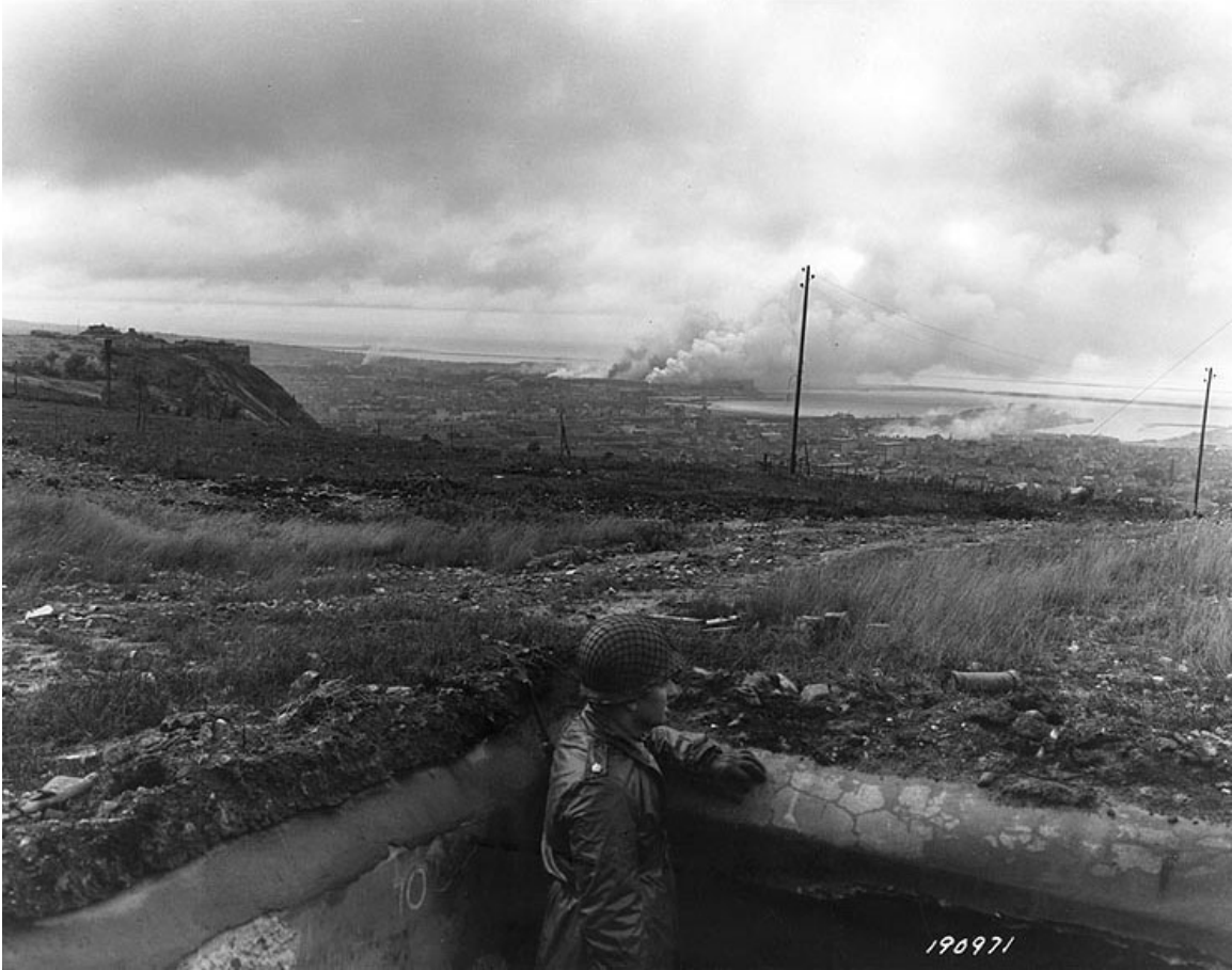
Figure 8. A US Army major looked over Cherbourg from one of the concrete pillboxes above the city, 26 June 1944
