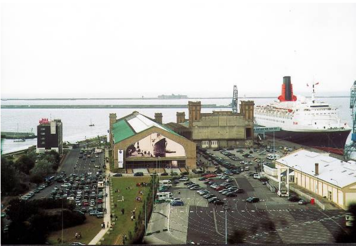
Figure 21. A view of the Cherbourg port liner terminal
