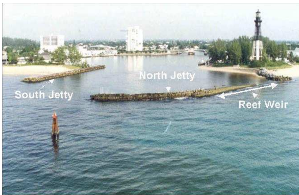
Fig. 5. Hillsboro Inlet, Florida, was the first sand-bypassing weir jetty system. The design incorporated a natural reef formation for the weir.
