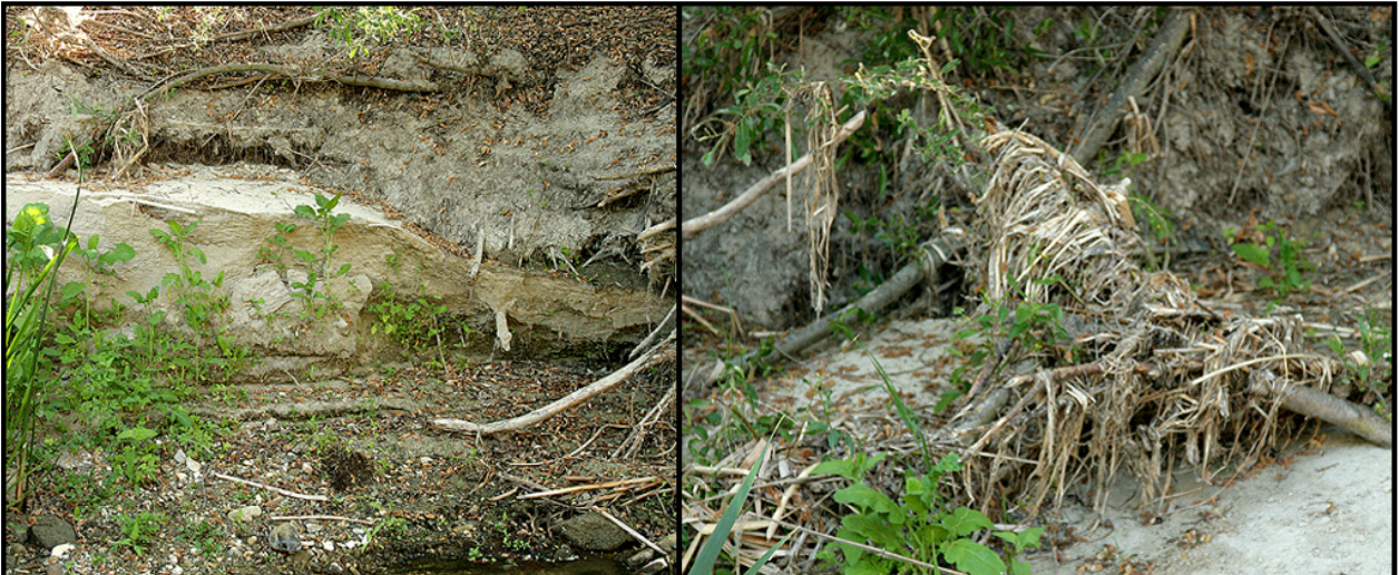
Figure 5. Shelving on the bank (left) and sediment deposits (right) were two features used to determine the OHWM.
