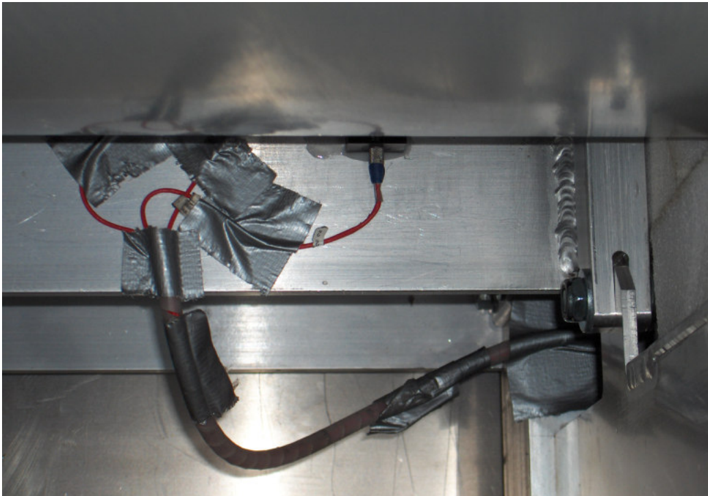
Figure 4. Placement of primary accelerometer on the central cradle support beam (looking down from above).
