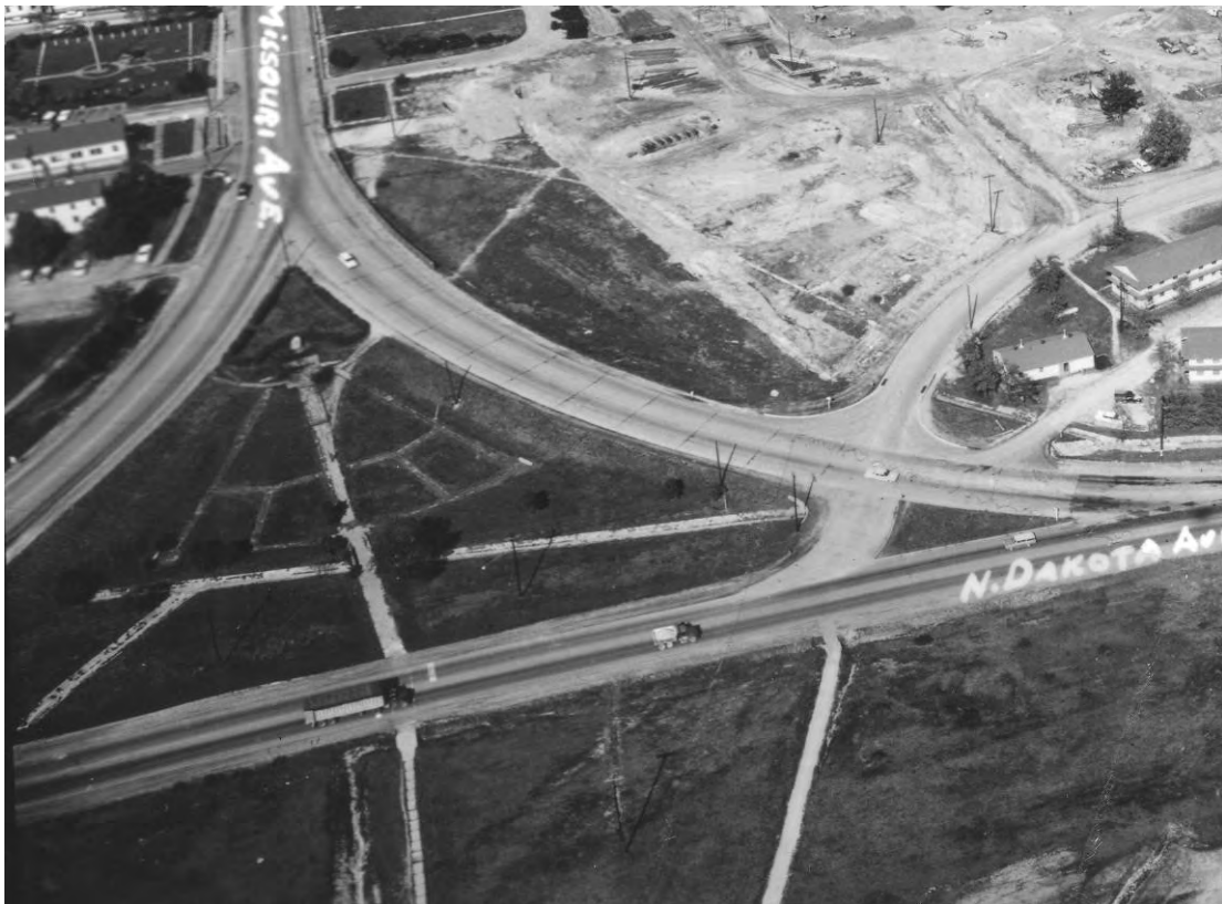
Figure 28. A low oblique photograph showing Veterans Park and construction on the new Health Center, October 1962 (NARA College Park, RG111-SC, photo 602 982).
