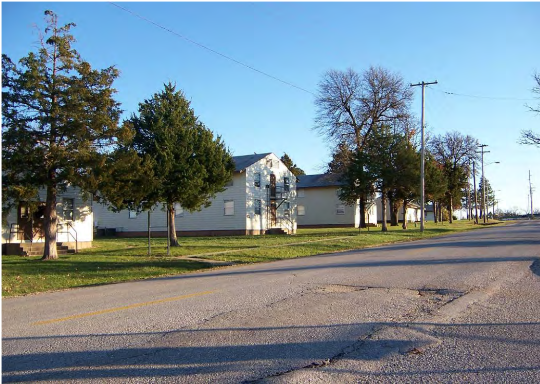
Figure 18. WWII temporary buildings used by the Missouri National Guard located in the southwestern corner of cantonment (ERDC-CERL, 2005).
