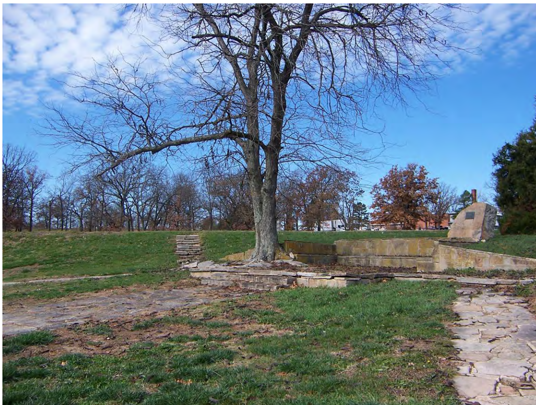
Figure 33. Veterans Park looking northwest at retaining wall, bench, and volunteer tree (ERDC-CERL, 2005).
