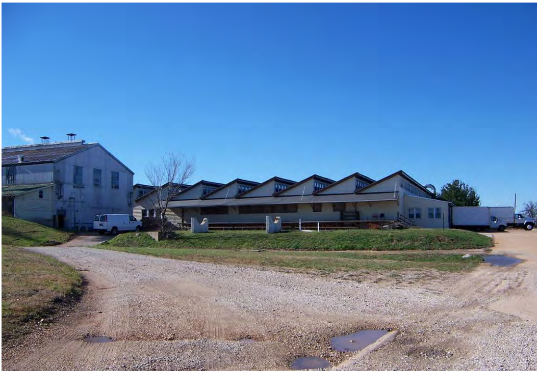
Figure 17. WWII-era laundry and steam buildings in warehouse area (ERDC-CERL, 2005).
