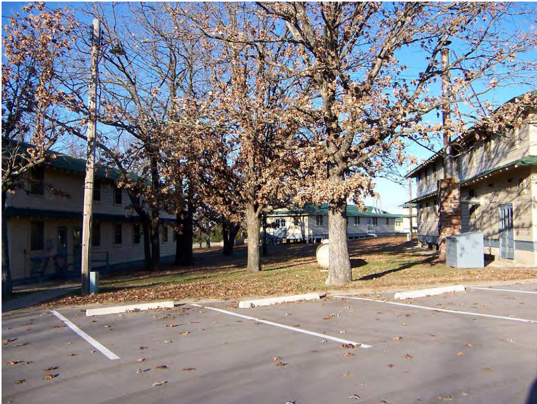
Figure 39. Photograph showing WWII temporary buildings built parallel to the contours (ERDC-CERL, 2005).
