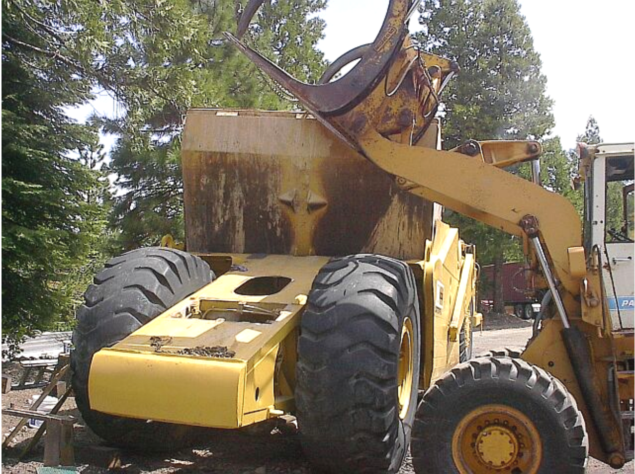
Figure 2: Removal of the Original Clamshell
