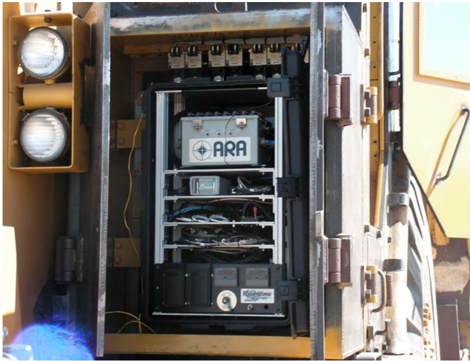
Figure 22: Telemetry Electronics - Vehicle
