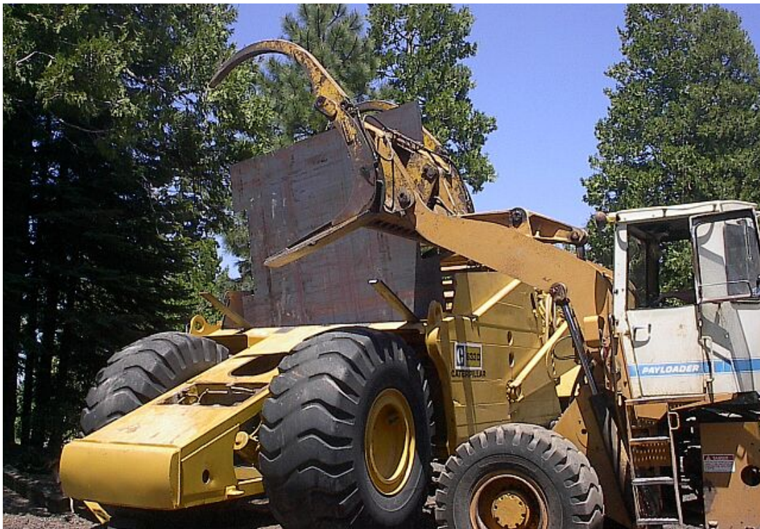
Figure 4: Backing Plate Installation - Ready for Screening Unit
