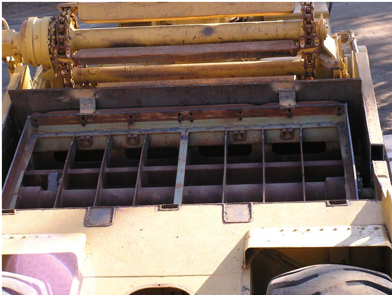
Figure 7: Screening Unit Installed Behind Backing Plate
