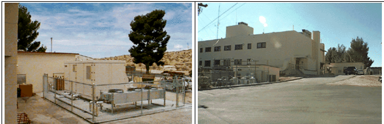
Figure 1. Fuel cell installation.
