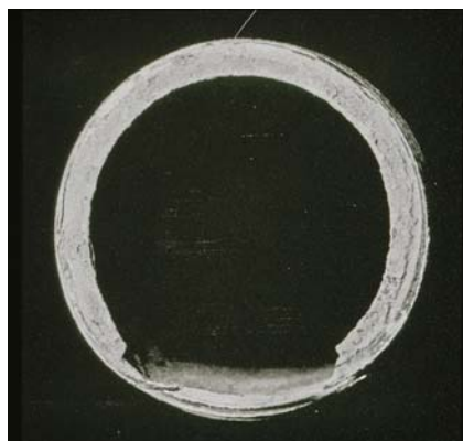
Figure 6. CO 2 attack of condensate return line.
