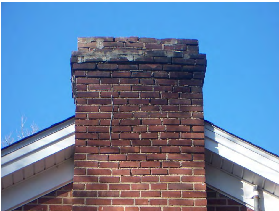
Figure 44. Soot staining, deteriorated mortar, and inappropriate brick reconstruction on kitchen addition chimney.
