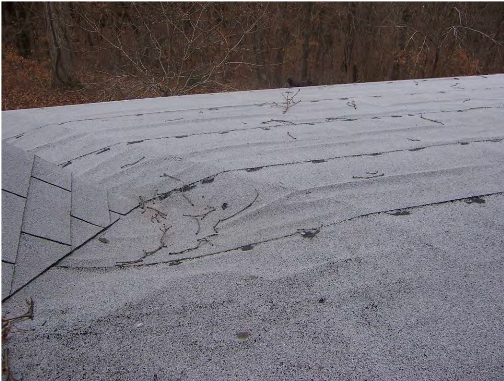
Figure 85. Incorrect connection between rolled asphalt roofing on screened porch and three-tab asphalt shingles.
