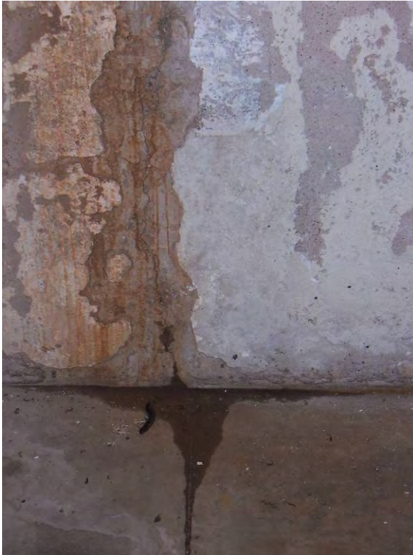
Figure 58. Water leaking into basement on east side crack after storm.
