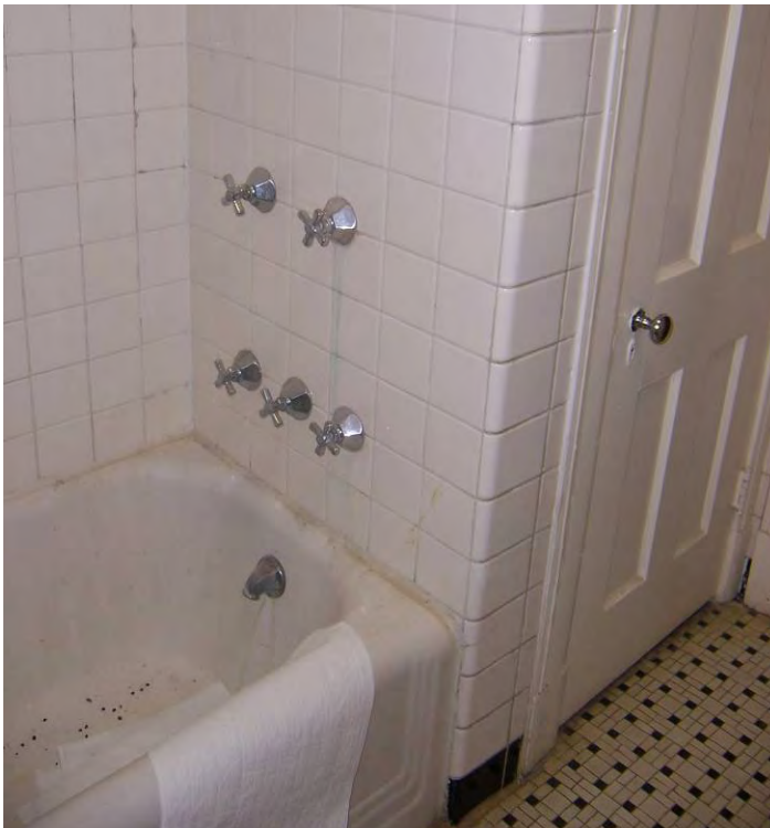
Figure 159. Original bathtub in first floor bathroom.
