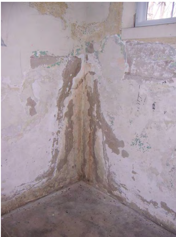
Figure 59. Northwest corner of northwest room in basement.
