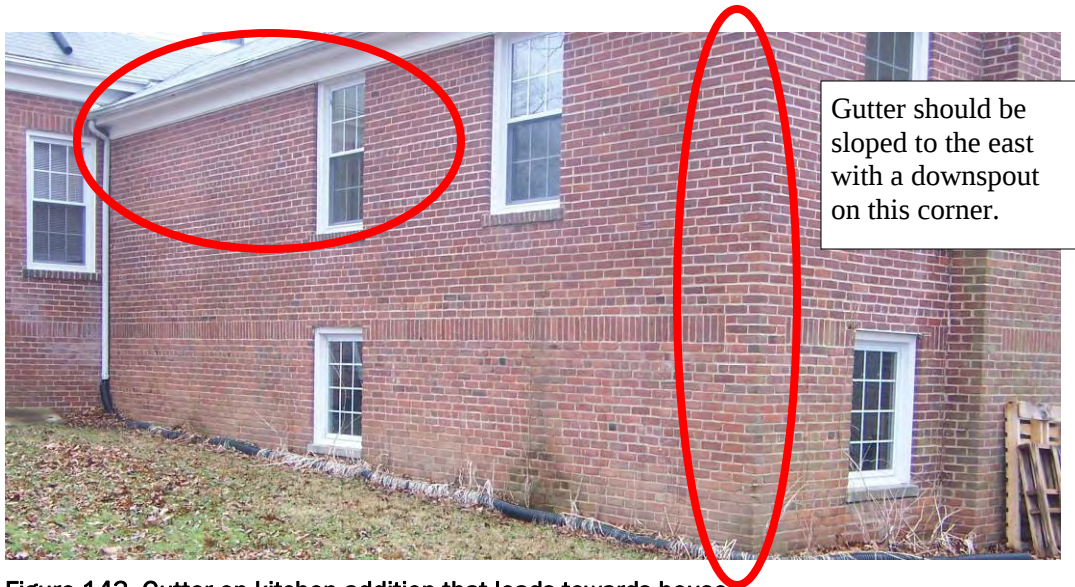
Figure 143. Gutter on kitchen addition that leads towards house.
