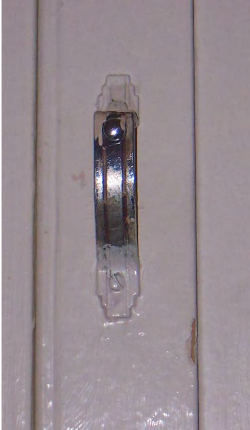
Figure 170. Original cabinet door pulls on hyphen cabinets.
