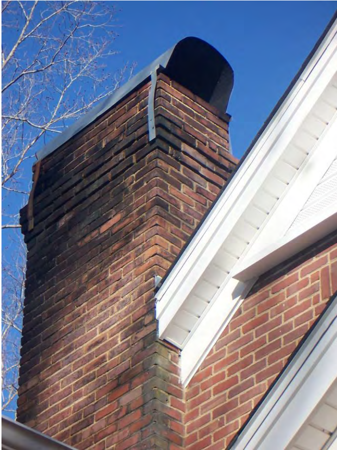
Figure 43. Closeup of soot staining and inappropriate chimney cap on south chimney.
