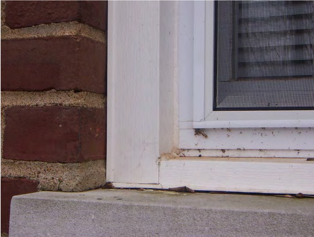
Figure 107. Closeup of aluminum covered window trim.
