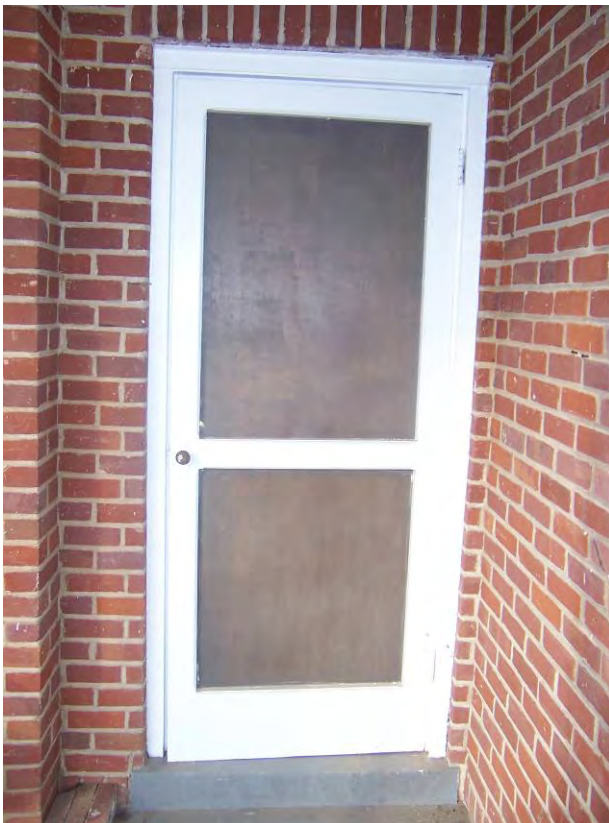
Figure 97. Wood screen door from screened porch to living room.
