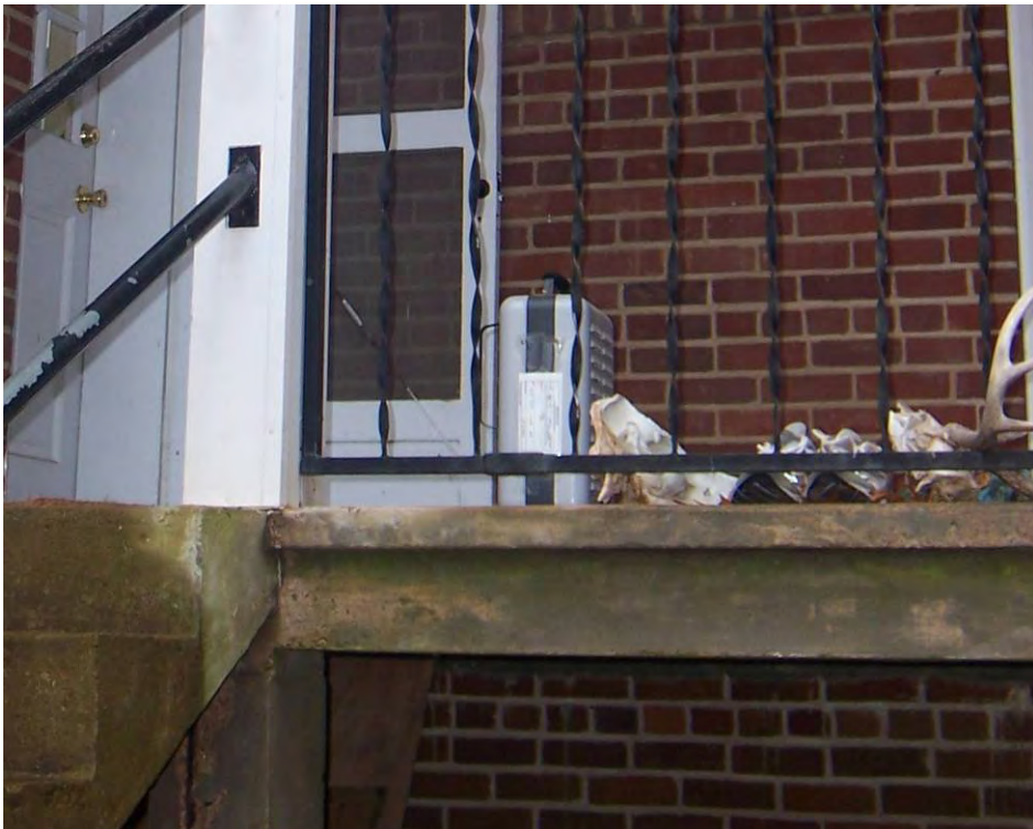
Figure 71. Closeup of concrete balcony.
