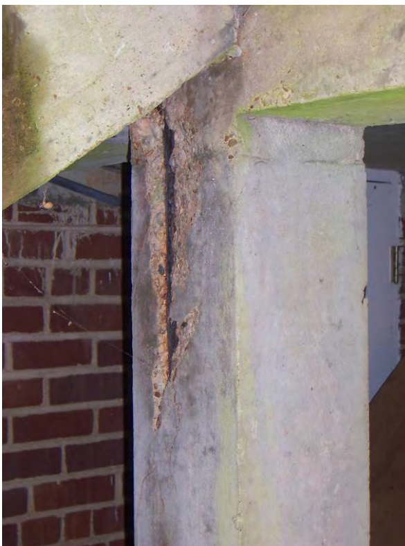
Figure 61. Closeup of spalled concrete pier with rebar subjected to weather.
