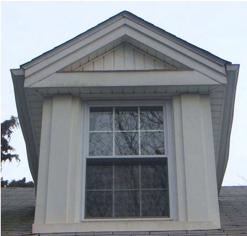
Figure 125. Metal covered decorative wood elements on dormer.
