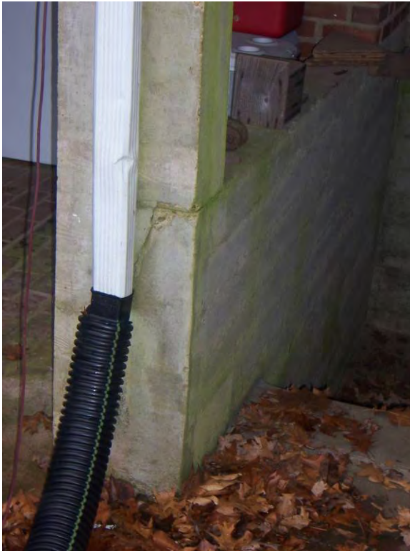
Figure 60. Concrete wall and concrete support pier with crack and lichen growth.
