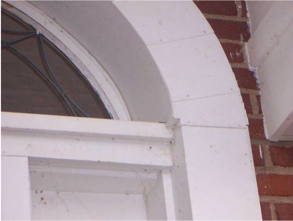
Figure 124. Metal covered decorative wood elements.
