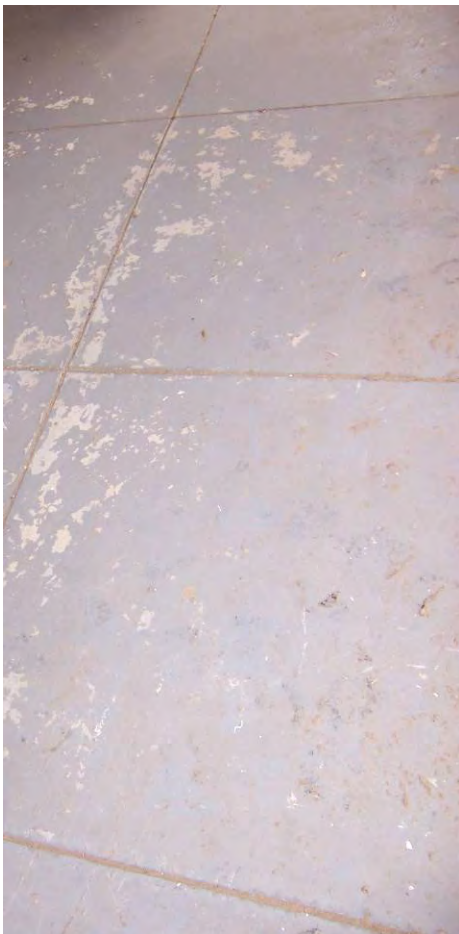
Figure 69. Flaking paint over concrete on screened side porch.
