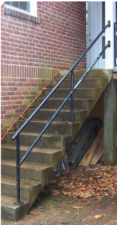
Figure 65. Steps up to kitchen entrance.
