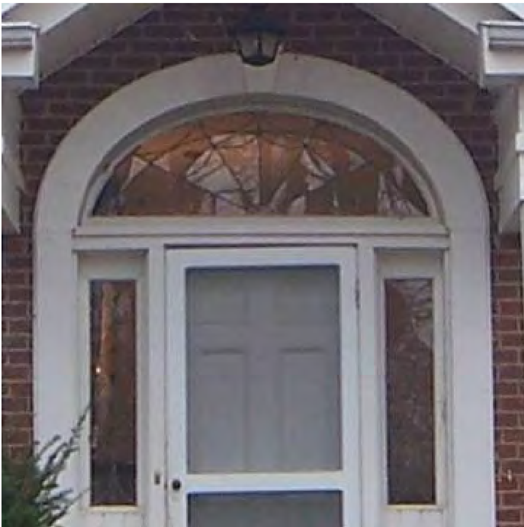
Figure 100. Aluminum covered wood sidelights and panels.
