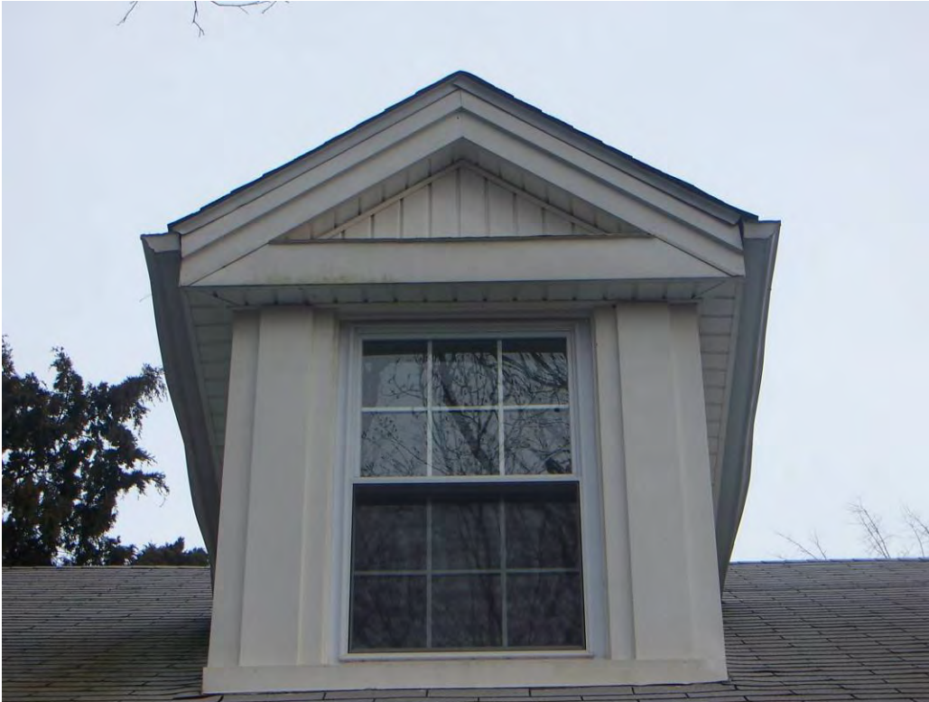
Figure 108. Closeup of replacement window and aluminum covered wood trim.
