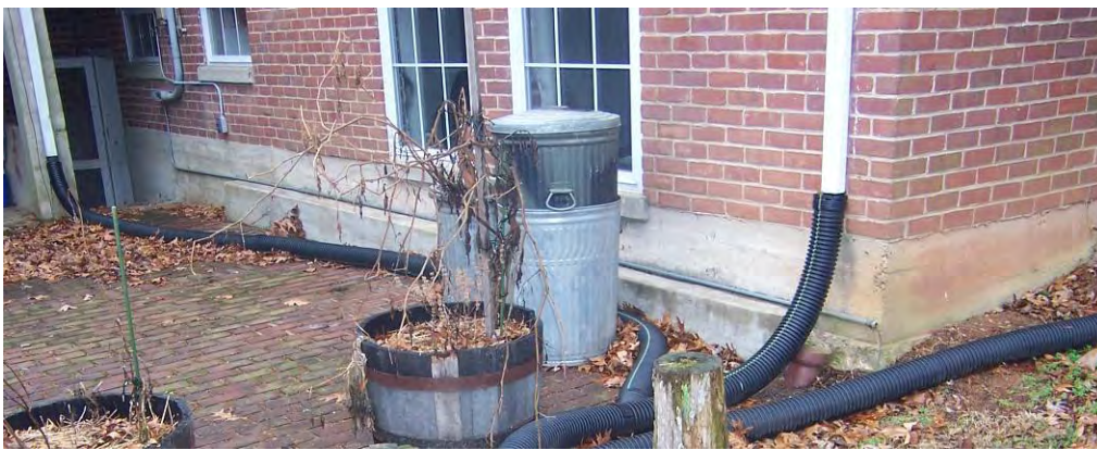
Figure 55. Example of concrete foundation on northeast corner.
