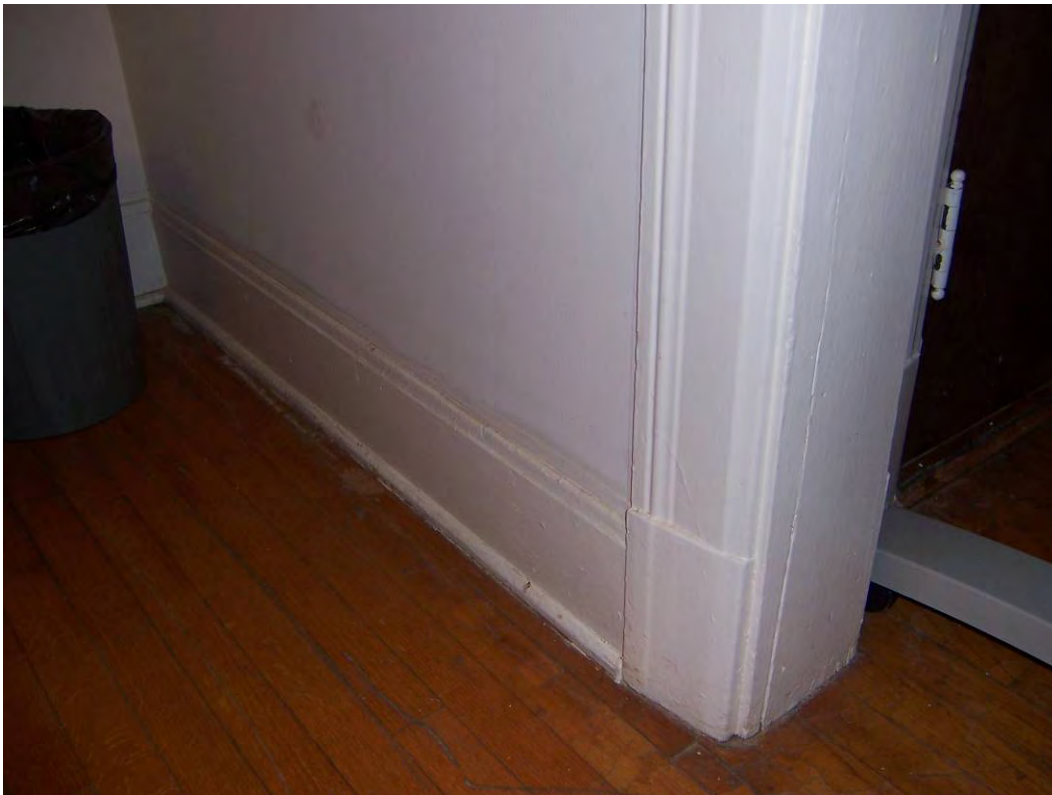
Figure 157. Millwork and floor in living room.
