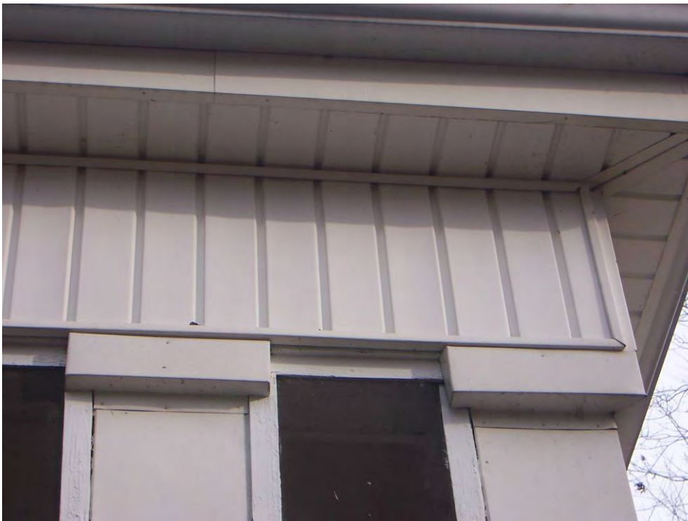
Figure 127. Metal covered decorative wood elements on screened porch.
