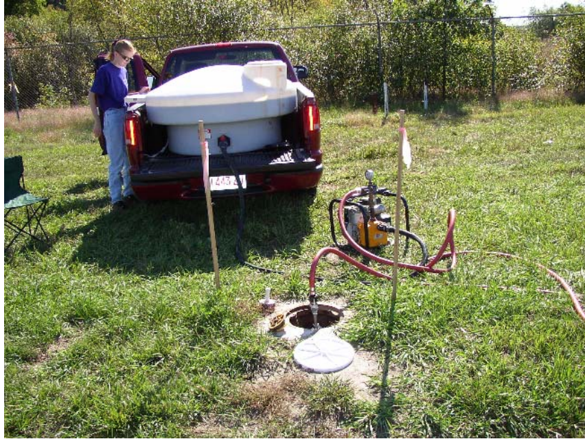
Figure 4. Reagent Mixing and Injection System Photograph—HAFB.
