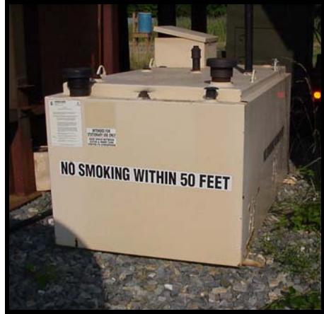
Figure 6. Shielded Diesel-Powered Generator and 500-Gallon Auxiliary Tank.
