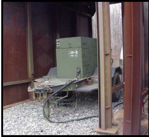
Figure 6. Shielded Diesel-Powered Generator and 500-Gallon Auxiliary Tank.
