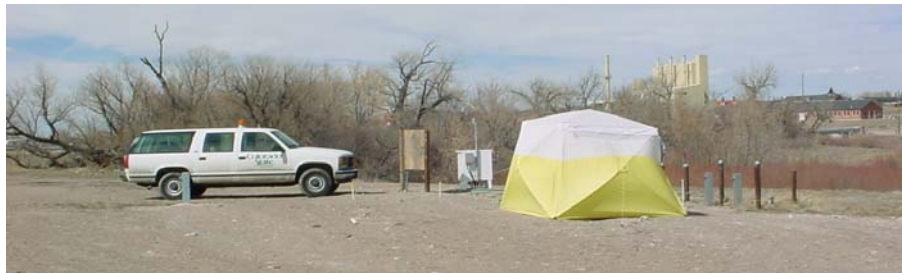
Figure 9. Final Grade Showing Sampling Shelter and Rectifier.
