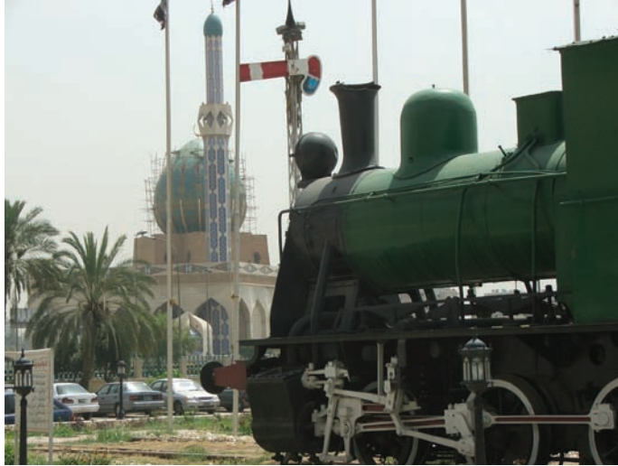
Baghdad Central Railway Station. SIGIR inspectors reviewed the renovations at this facility in Summer 2006.
