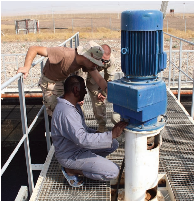
U.S. and Iraqi engineers inspect the broken sweep arm at the Al Kasik Waste Water Treatment Plant.
