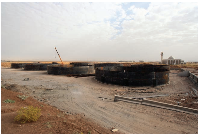
Site Photo 10. Overall progress of water storage tank construction, as of August 1, 2006.
