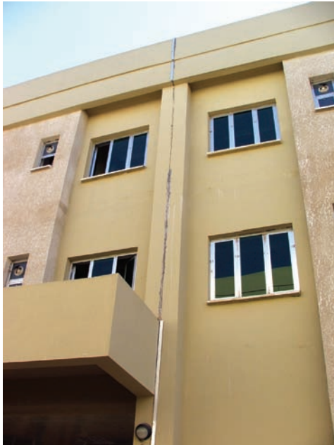
Site Photo 24. Exterior expansion crack on the instructor barracks.
