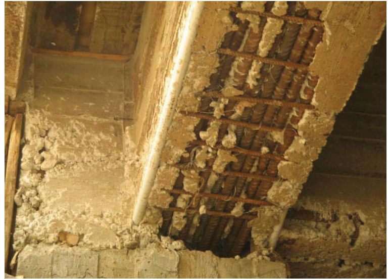
Site Photo 25. Evidence of improperly placed exposed reinforcement bar, PVC conduit, and rust.
