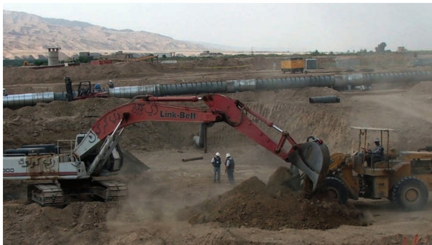
Pipeline construction in northeastern Iraq.
