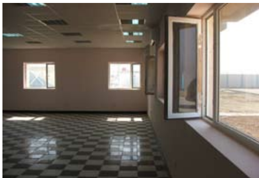
Dining facility inside barracks
