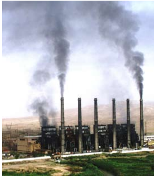
Baiji Power Plant
