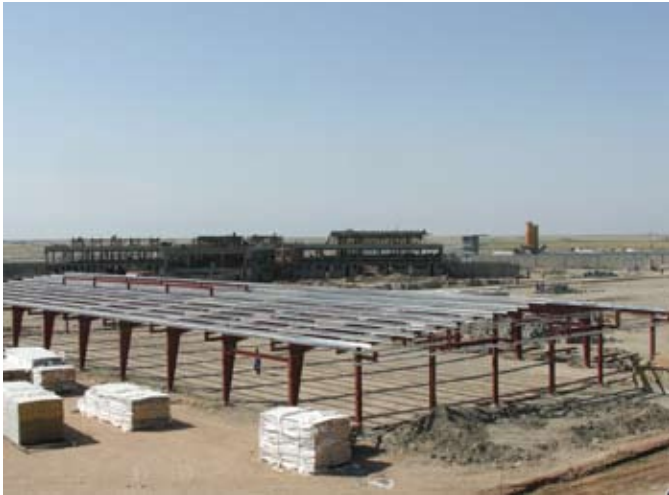
Kitchen and laundry building structural frame
