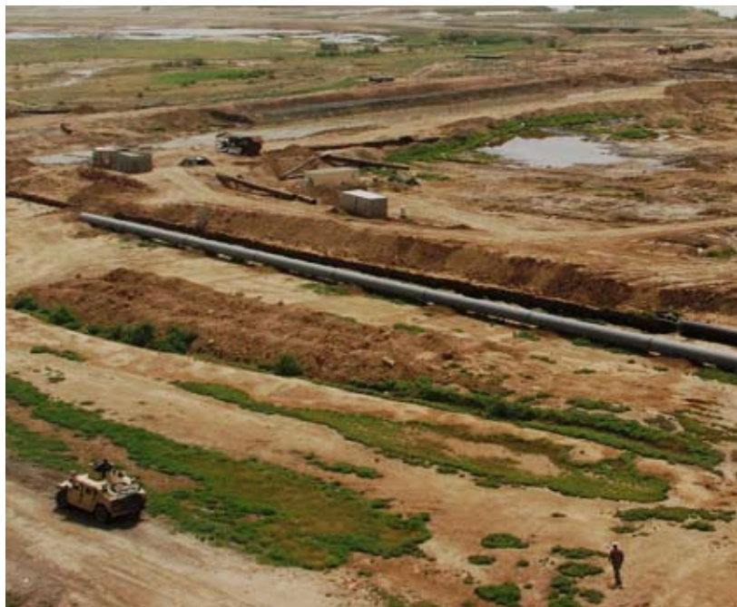
Welded pipe string at the Zegeton Canal
