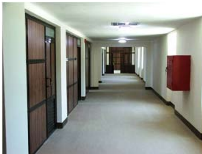
View of new interior partitions
