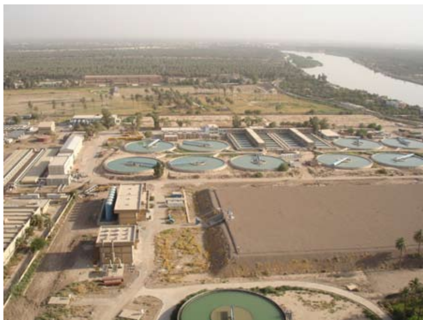
Shark Dijlah water treatment plant, second largest in Baghdad
