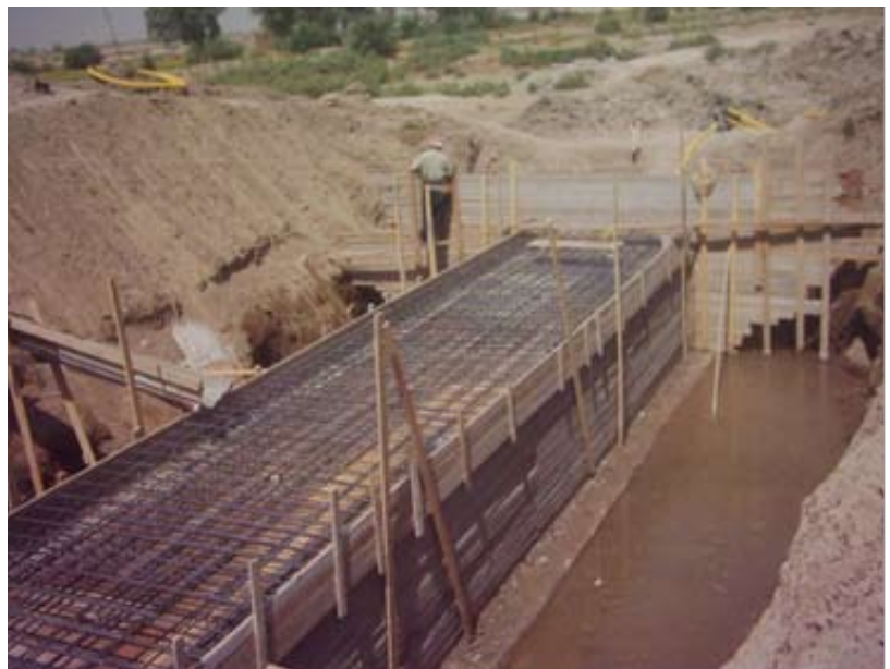
Construction of a box culvert (photo provided by USACE)
