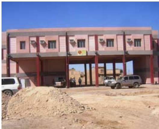
Exterior view of the front of the fire station (photo provided by USACE)
