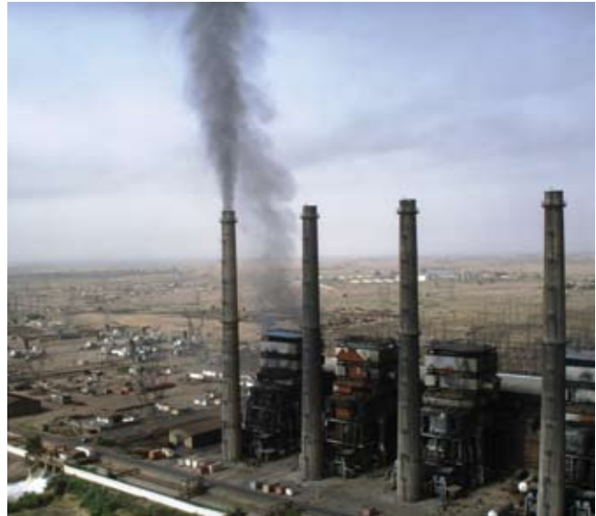
The Baiji Power Plant is a major producer of electricity for Iraq.
