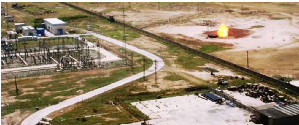
Gas being flared at an oil facility
