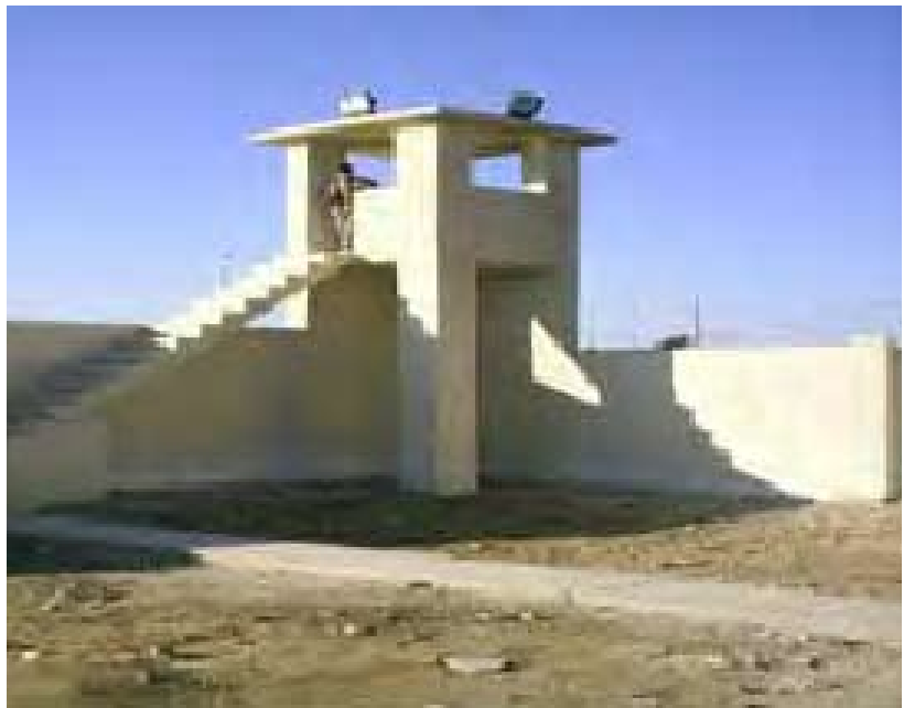
Corner guard tower with perimeter wall of police station
