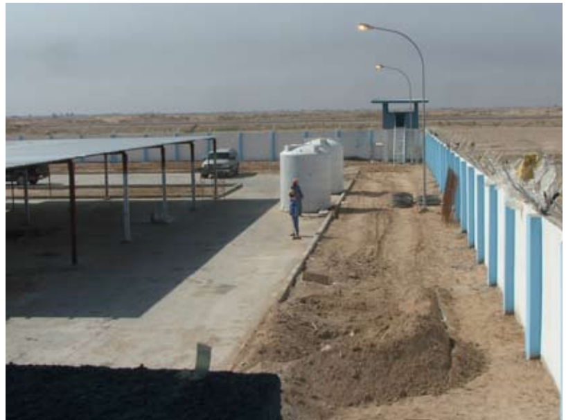
Light poles, perimeter walls, and covered parking area
