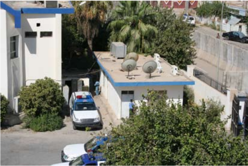
Site Photo 17. Only two (left rear edge of rooftop) of six split-unit air conditioners required were installed in the new reception center.
