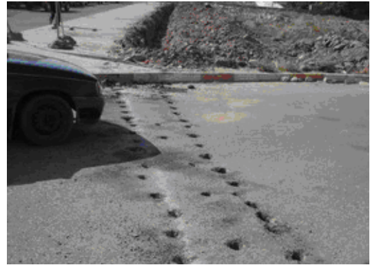
Site Photos 23 and 24. Hard surface break-up equipment in preparation of material removal. (Photos provided by USACE)
