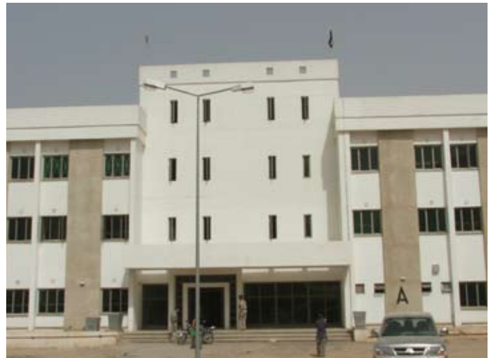
Site Photo 30. Outside view of new cadet barracks building.
