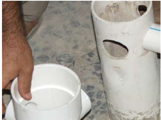
Site Photo 36. Contract-specified wastewater pipe connection is shown on the lower left.
