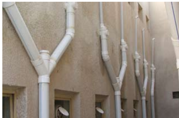
Site Photo 9. Reworked drain lines with upgraded material and improved "Y" design.
