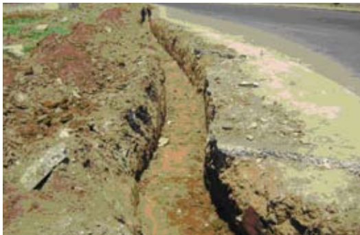
Site Photos 25 and 26. After the trench was excavated and the base compacted (left), the cable was positioned on a sand layer (right). (Photos provided by USACE)
