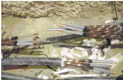
Site Photos 27 and 28. Cables were spliced together with splice kit (left), and heat was applied (right) to shrink outer cover used to protect cable splice. (Photos provided by USACE)
