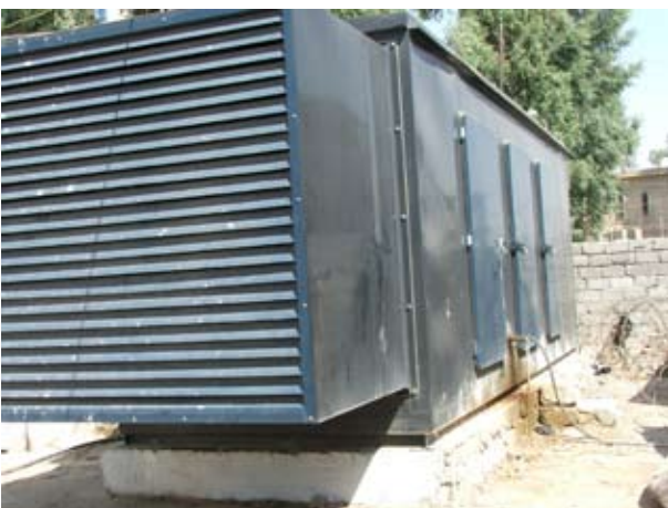
Site Photo 19. Final site where generator was placed by Iraqi Police (IP).
