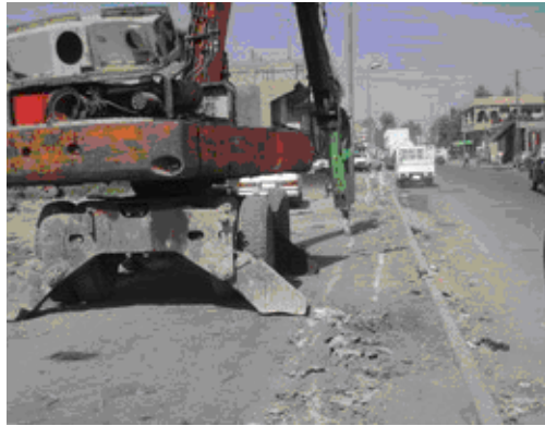
Site Photos 23 and 24. Hard surface break-up equipment in preparation of material removal. (Photos provided by USACE)
