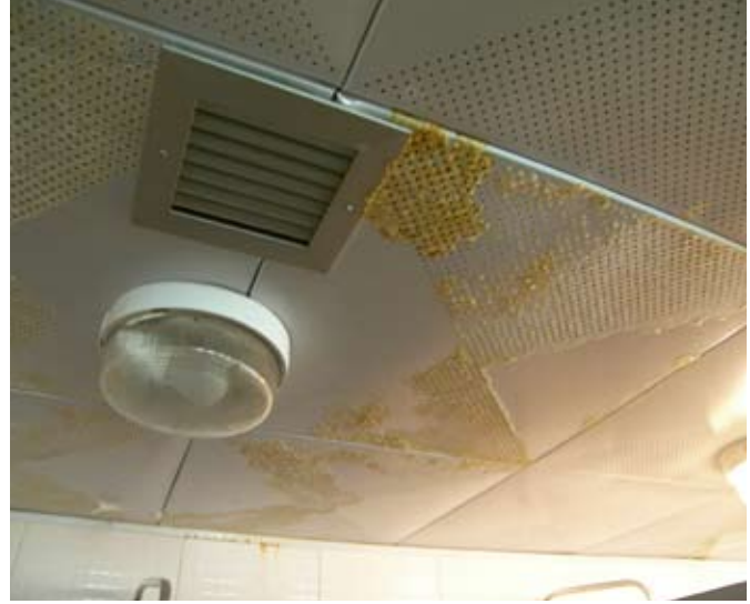
Site Photo 34. Crystallized urine on ceiling tile.
