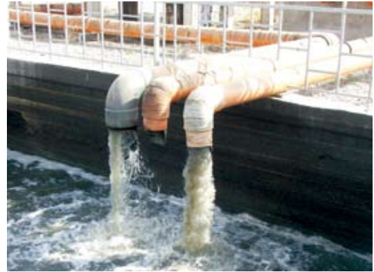
Al Kasik Water Treatment Facility
