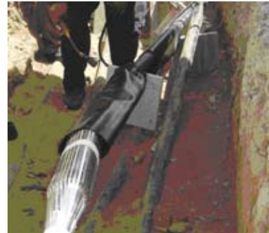
Site Photos 27 and 28. Cables were spliced together with splice kit (left), and heat was applied (right) to shrink outer cover used to protect cable splice. (Photos provided by USACE)
