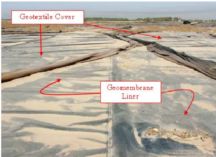
Site Photo 4. Exposed geomembrane liner.
