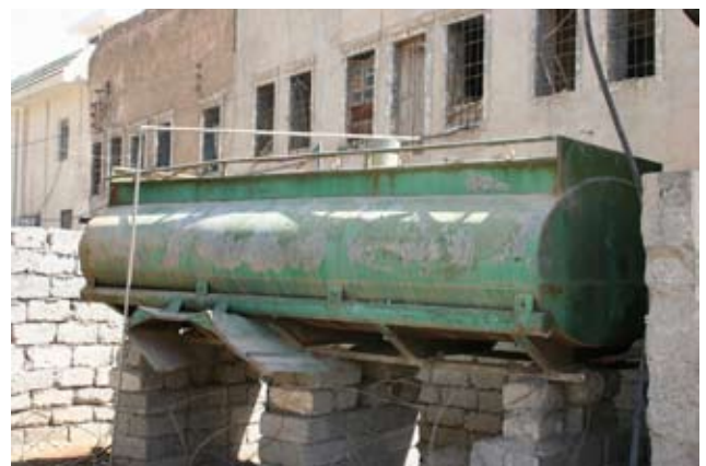
Site Photo 20. Old fuel truck tank placed by IP to supply the generator.
