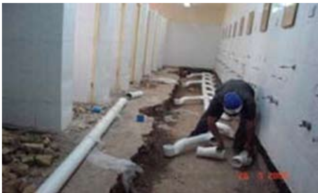
Site Photo 8. Extensive rework was required in dormitories to install watertight plumbing fittings. (Photo courtesy of ECCI)
