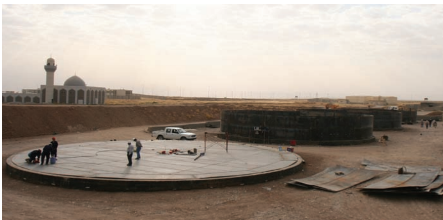
Water storage facility at the Al Kasik Military Training Base
