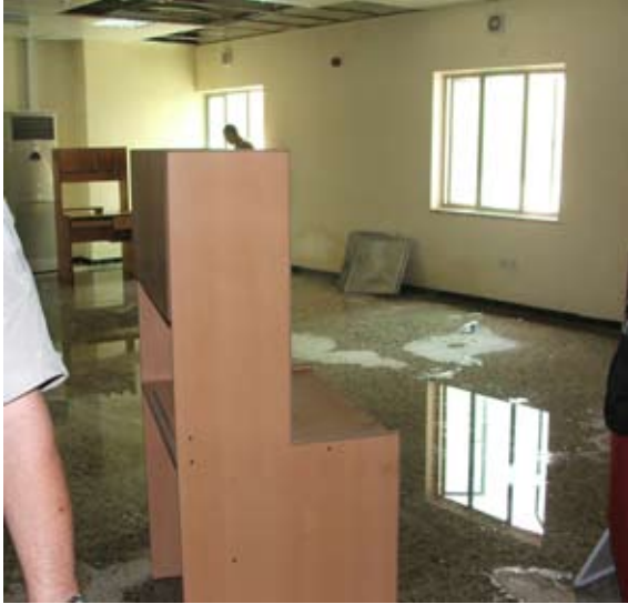
Site Photo 33. Water damage from leaking ceiling.
