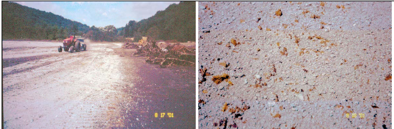
Figure 8. Applying waste paper fiber in Area 3b. Figure 9. Cover of waste paper fiber over bony coal mine residue in Area 3a.
