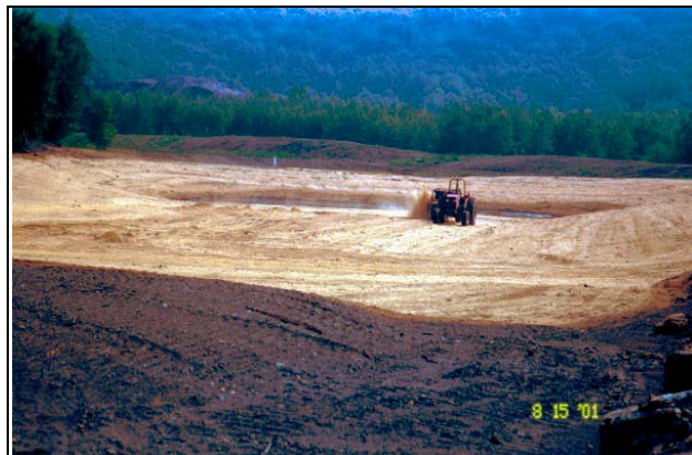
Figure 4. Sawdust application to wetland Areas 1a and 1b.
