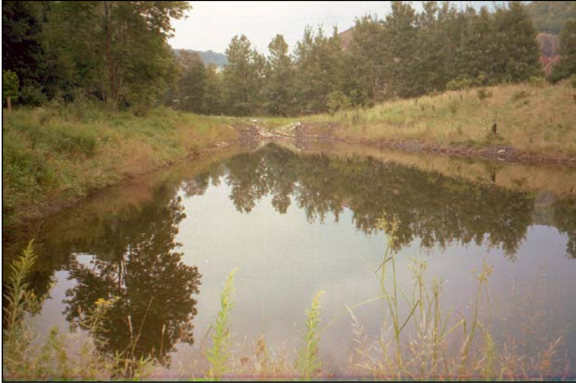
Figure 11. Acid mine drainage passes through Pond 1, the first of six lime treatment ponds (Figure 1).
