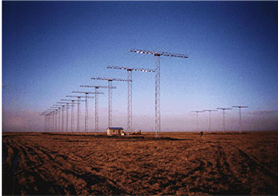
Figure 29. The Antenna Element of OTHR Radar (From [34]).
