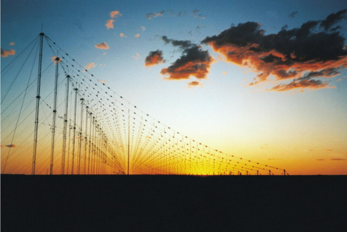
Figure 12. The JORN Transmission Antenna Array (From [15]).
