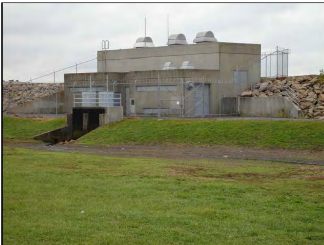
Figure 33. Clark Cove pump station, operated by City of New Bedford. Grassy field in foreground serves as temporary storage after heavy rain.
