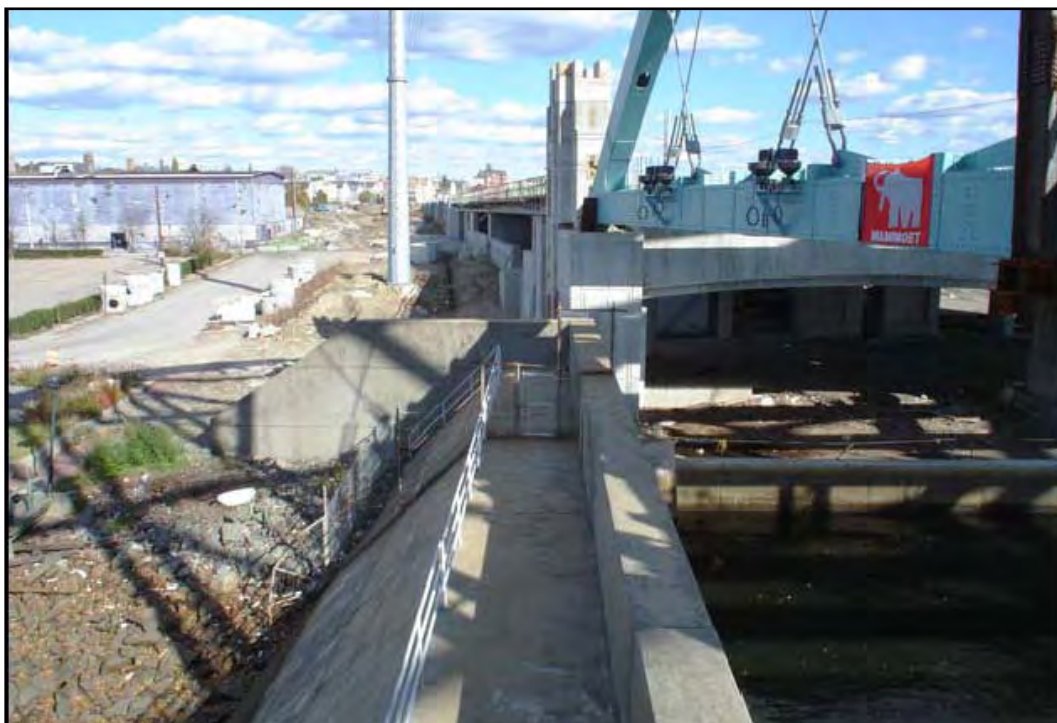
Figure 18. View east from Fox Point hurricane barrier showing ramps and newly-built I-195 bridge, 4 November 2006. Concrete freeway ramps substitute for some of original dike.
