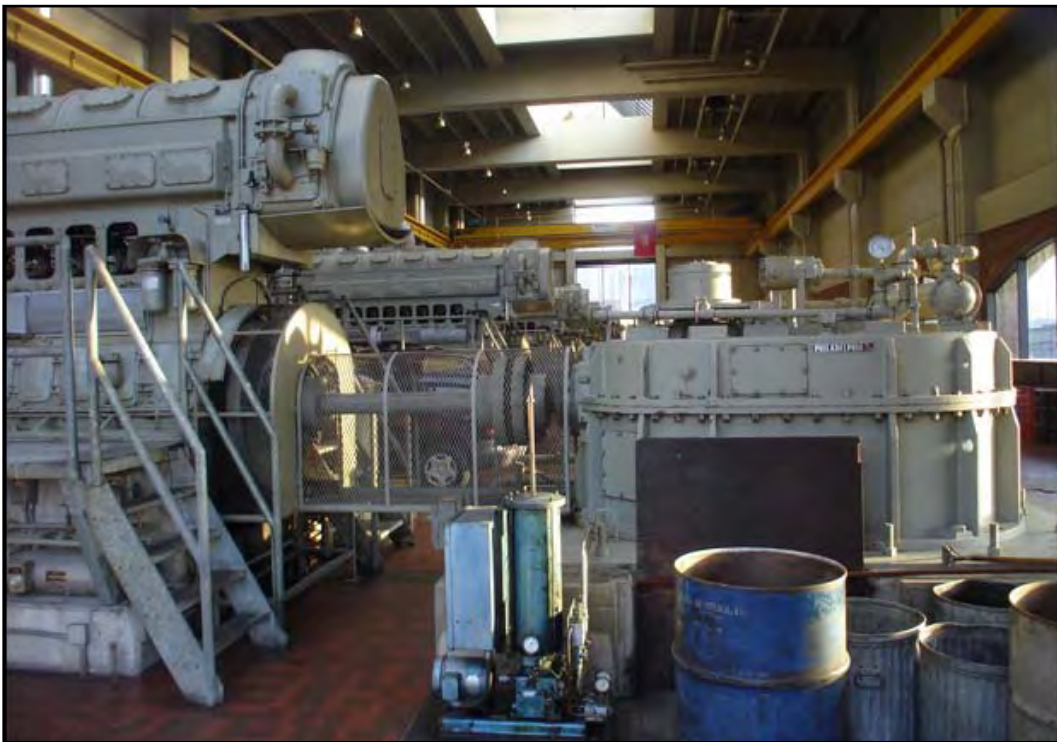
Figure 52. Diesel engines and pumps in Charles River Dam, 1 November 2006.
