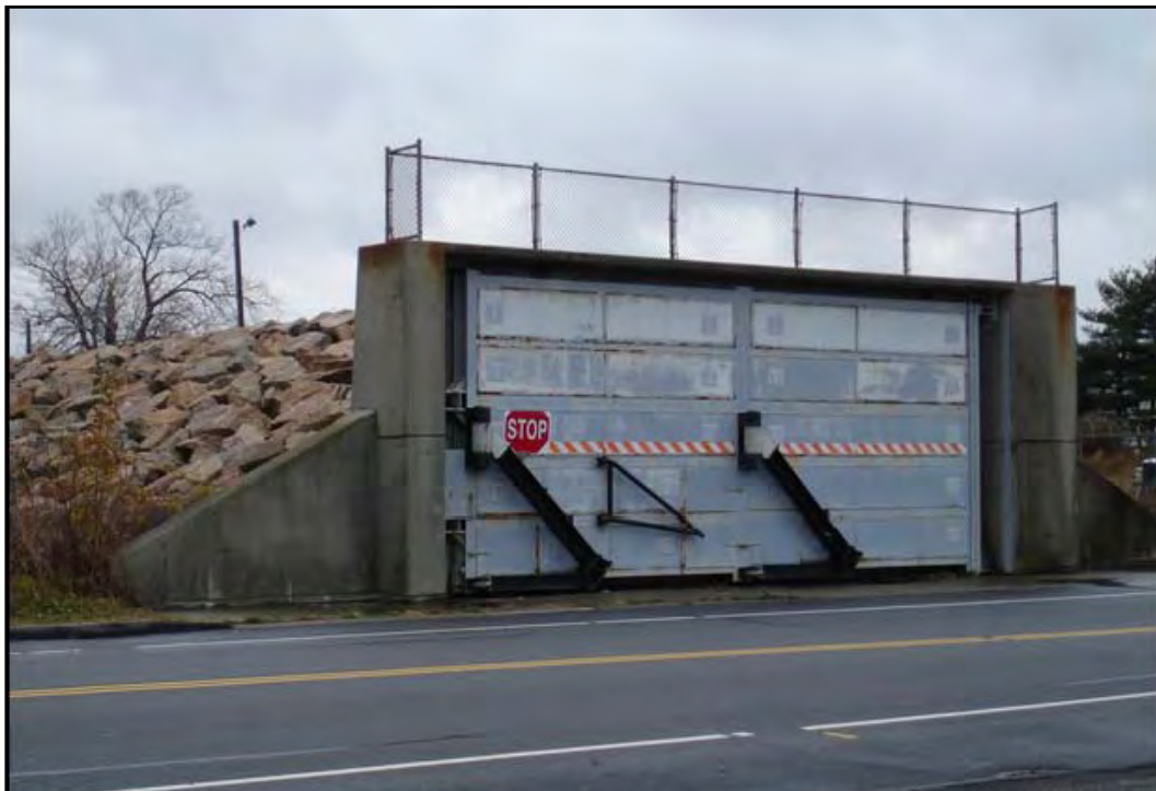
Figure 32. Steel swing gate at E Rodney French Boulevard, New Bedford.
