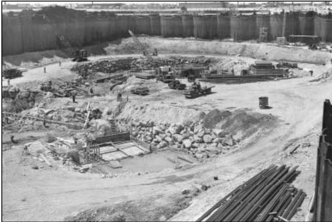
Figure 23. Sector gate foundation work within protective cofferdam, 5 May 1964 (photograph courtesy of New England District).
