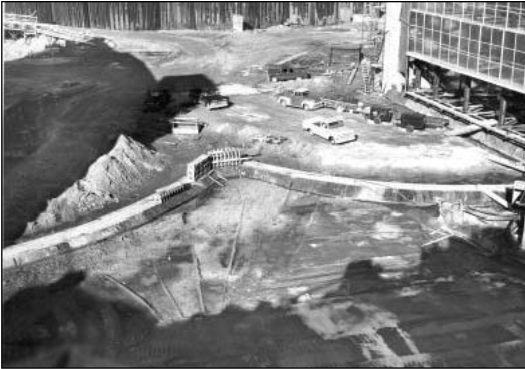
Figure 25. Construction of guide for sector gates, 16 December 1964. Trucks show scale of this project (photograph courtesy of New England District).
