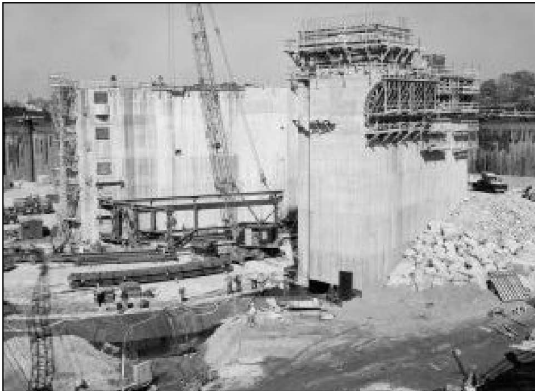
Figure 27. East sector gate steel erection, 15 October 1964 (photograph courtesy of New England District).
