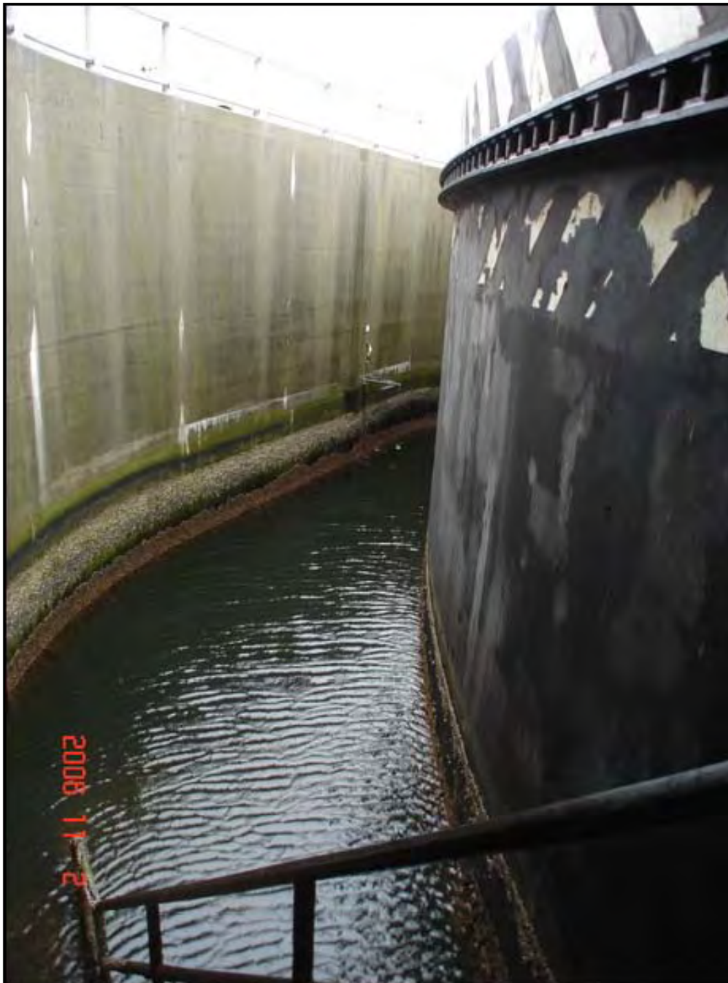
Figure 31. West side section gate in its well. Cogs near top of gate are engaged by teeth of opening mechanism. Silt builds up in well and has to be flushed with compressed air, but gates are often difficult to fully retreat.
