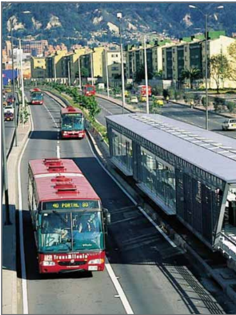
Figure 34. The Transit Boulevard: Linking New Neighborhoods. Along the proposed boulevards, the emerging transit mode known as Bus Rapid Transit (BRT) would offer low construction cost, short construction time, capacity for phased implementation, operational flexibility, and effective transit service. In some cases, Light Rail Transit (LRT) may be a viable alternative. The transit service then supports the development of new neighborhoods flanking the boulevards. Residents would generally live no further than a 15-minute walk from the boulevard.
