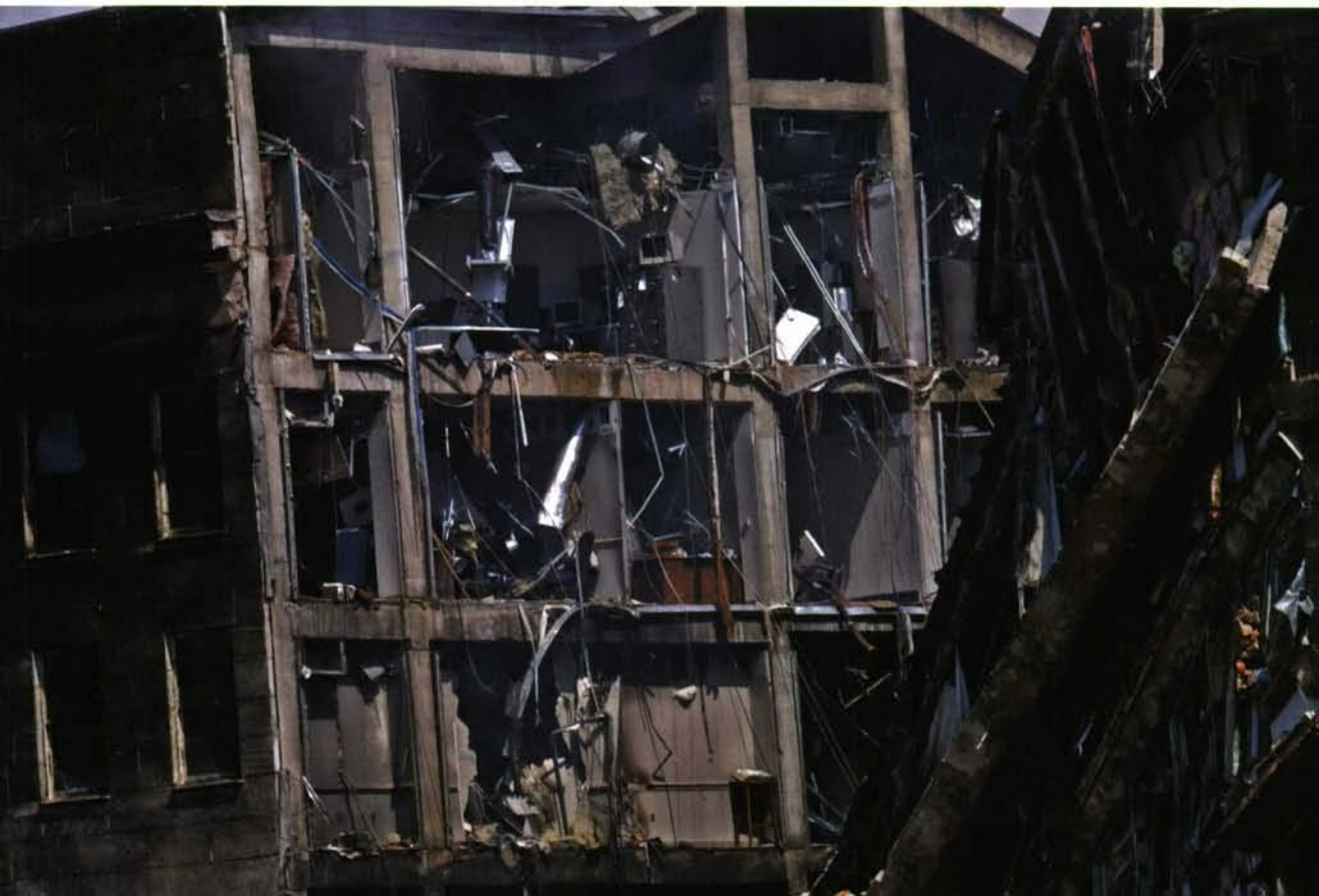
Damaged interior offices sheared open by the collapse of the E Ring.
