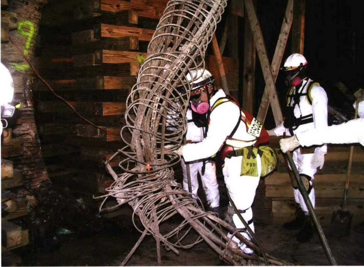
Above: Removing a damaged building column. Below: Weary workers emerge from Heliport entrance.
