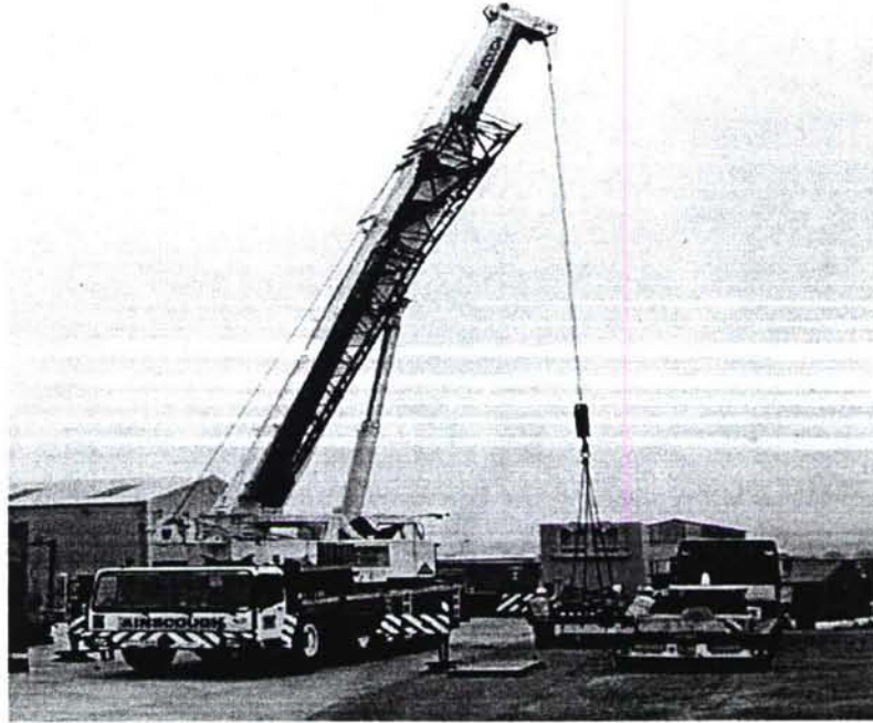
Figure 3-1. TC-60 Detonation Chamber Being Unloaded
