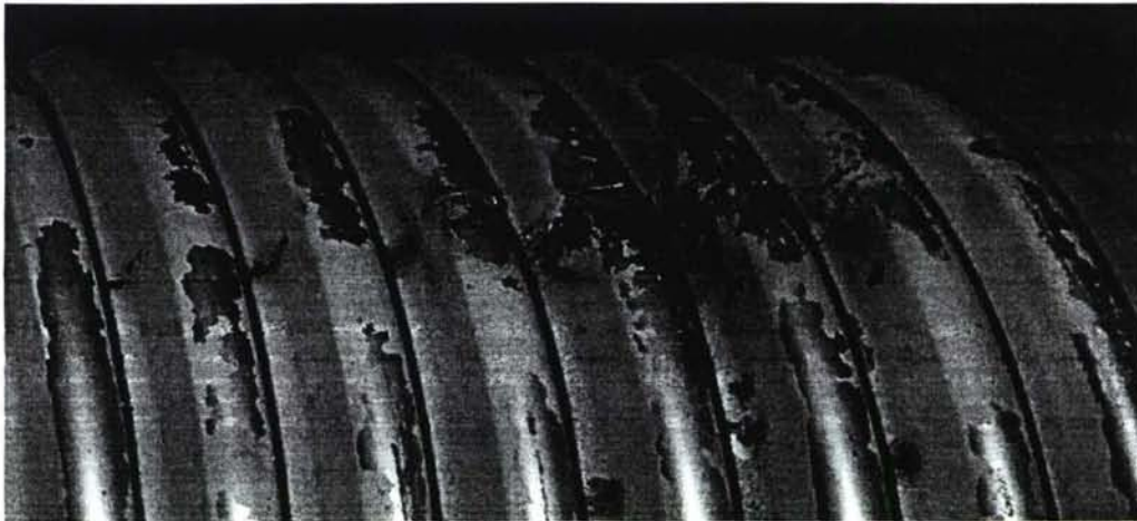
Figure 5-1. Cracked Expansion Joint
