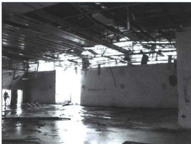
One of the numerous damaged buildings at Forward Operating Base Speicher that was infested with birds. Portions of the interior of this building were being renovated for use. Numerous openings made exclusion of birds impossible.
