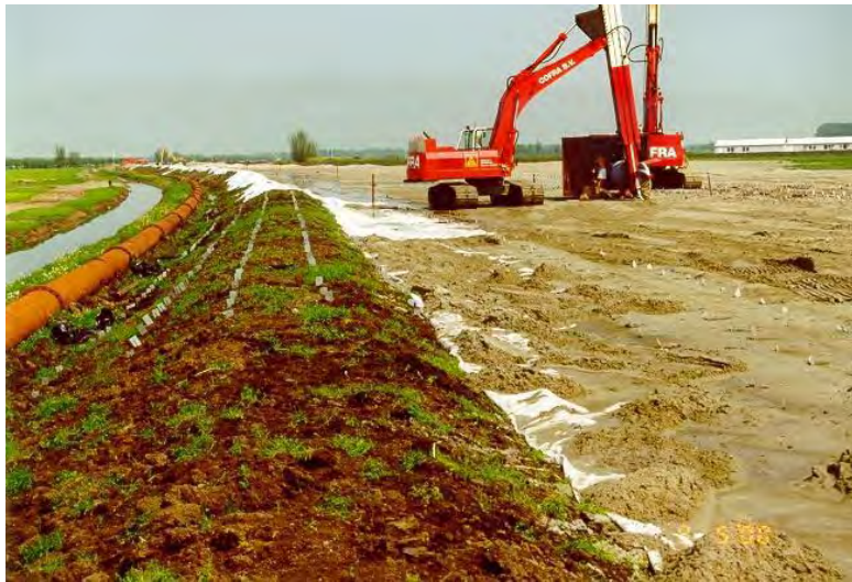
Figure 120 Inserting vertical strip drains to decrease pore pressure
