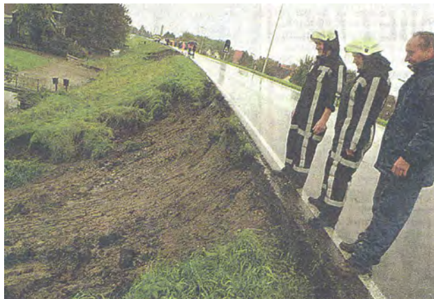
Figure 118 Levee near Hook of Holland, Netherlands, with steep slope landside, silty material, after heavy rainfall. Newspaper photo.
