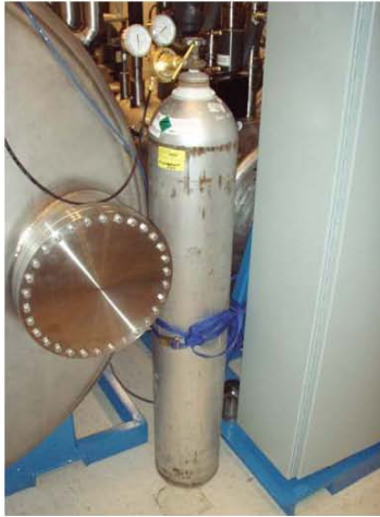
Figure 21: Gaseous Nitrogen Source
