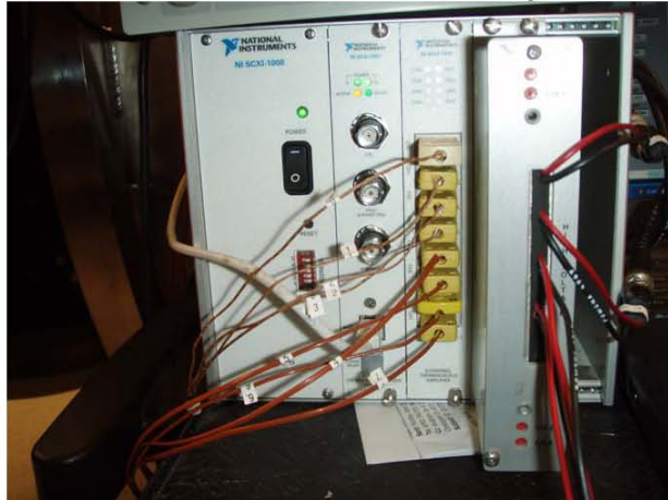
Figure 31: Connection of Thermocouple and RTD Wires to Wiring Interface on Data Acquisition System
