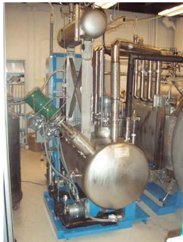
Figure 16: Thermal Control Unit (TCU)
