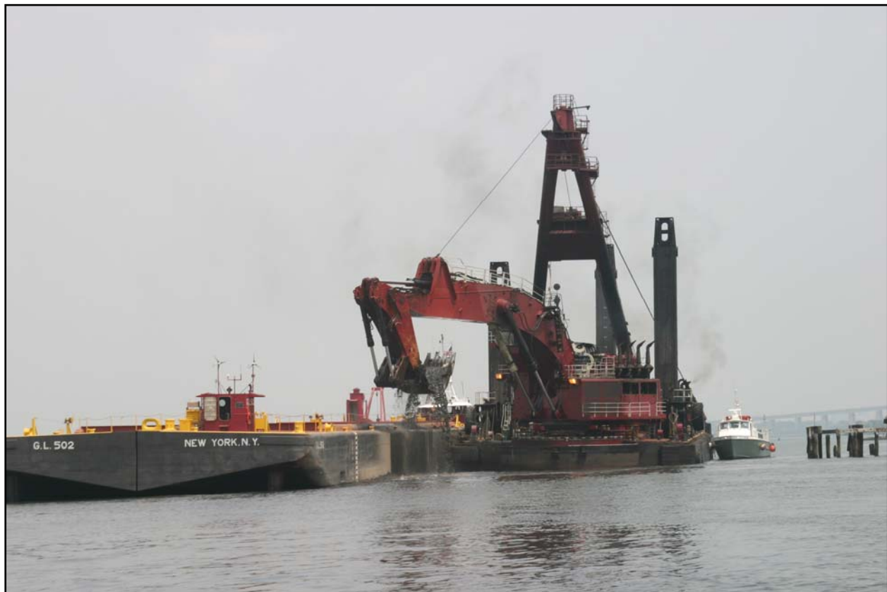
Figure 7. Backhoe Dredge (Dredge New York, courtesy of Great Lakes Dredge and Dock Company).
