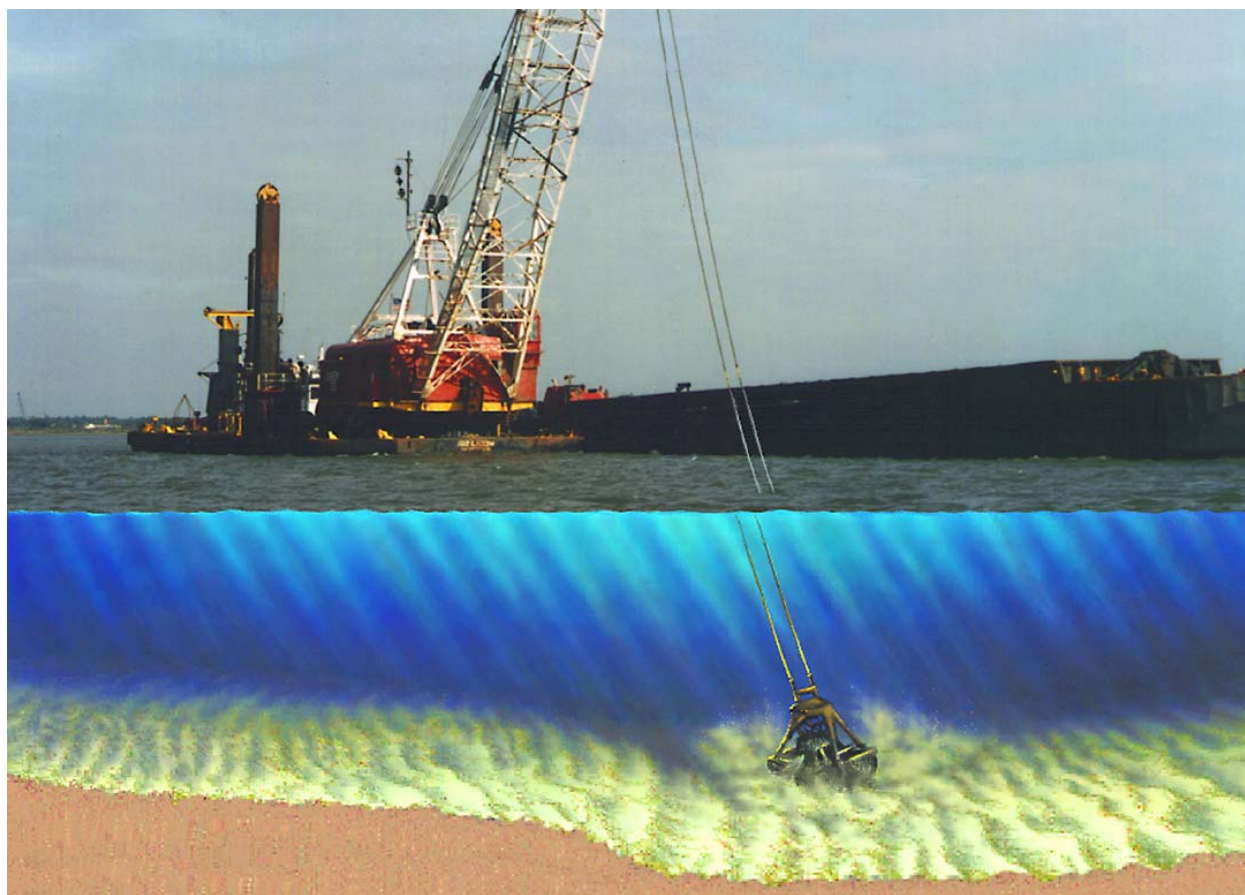
Figure 2. Clamshell (bucket) dredge.
