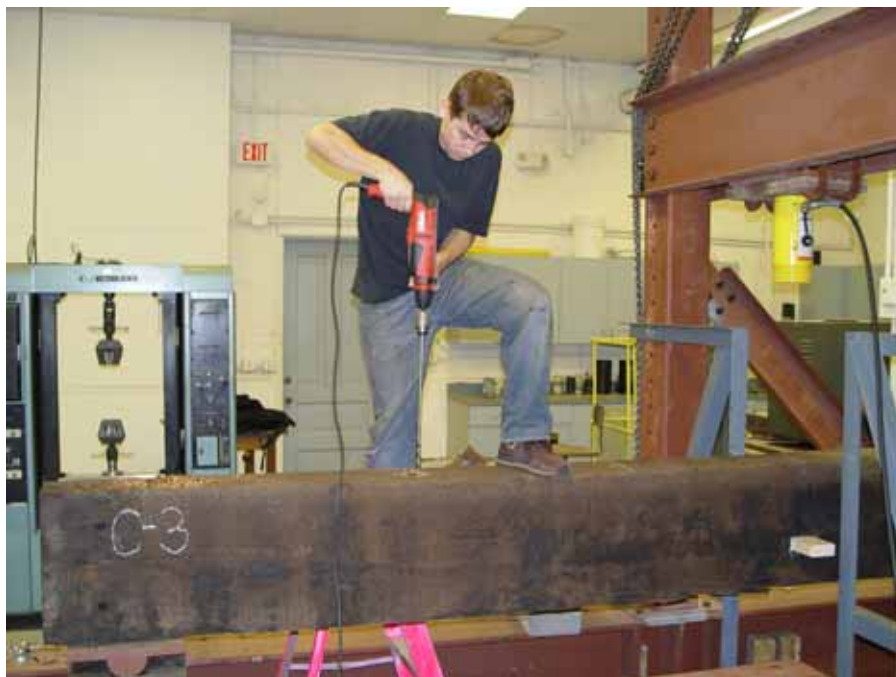
Figure 35. Holes being drilled with TE 2.
