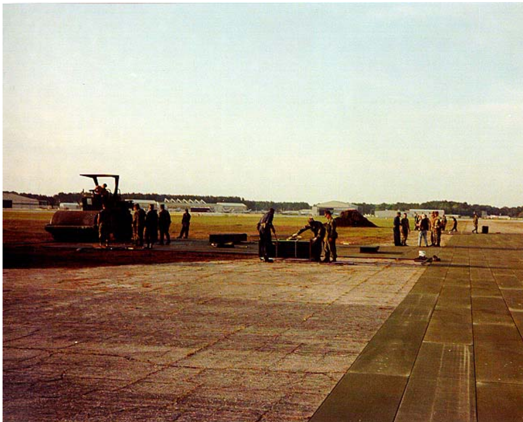
Figure 1: AM-2 matting being assembled
