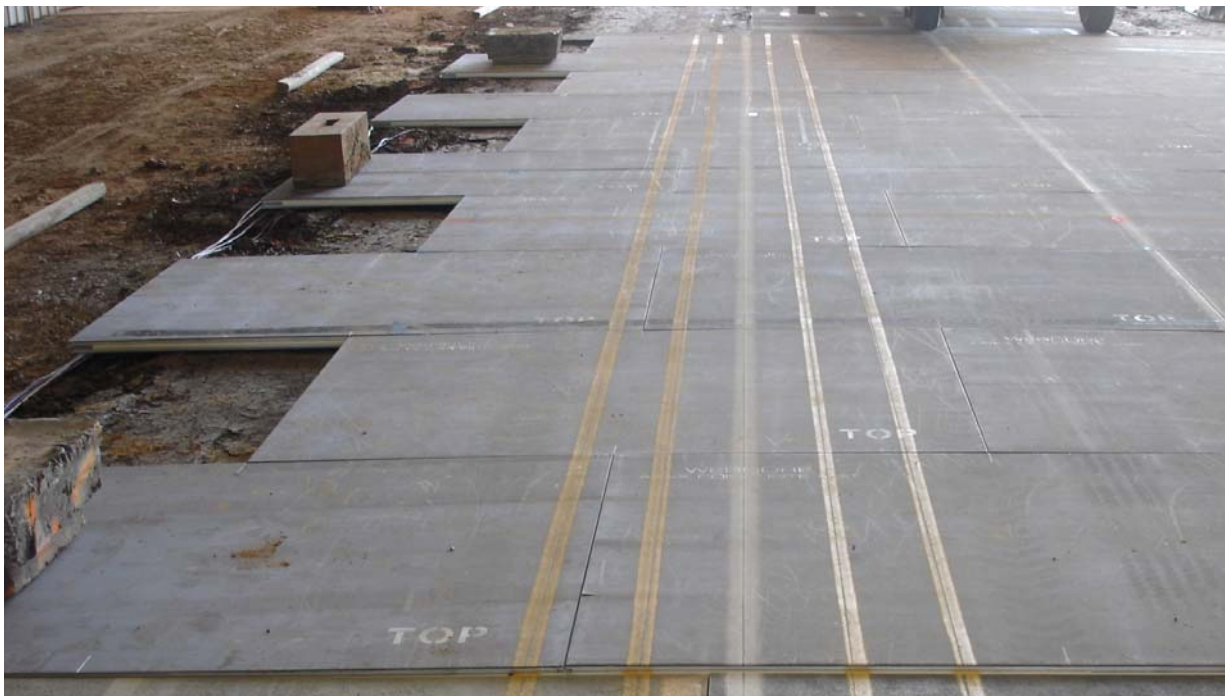
Figure 20: Composite AM-X mat layout with traffic lanes and weighted edges.
