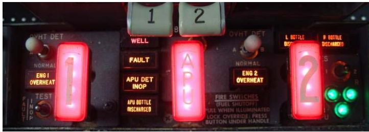
(Photo of cockpit fire panel above is from the “737 web site” and used with permission by its author, C. Brady.)
