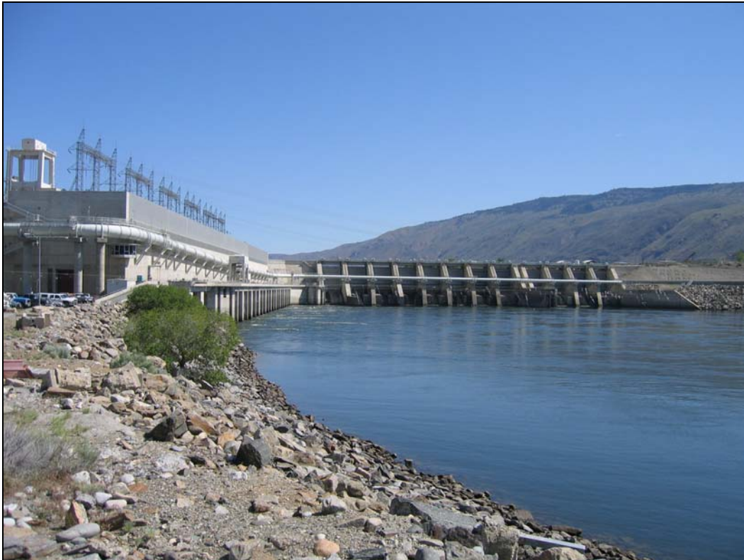
Figure 5. Rocky Reach hydroelectric project operated by the Chelan County Public Utility District.
