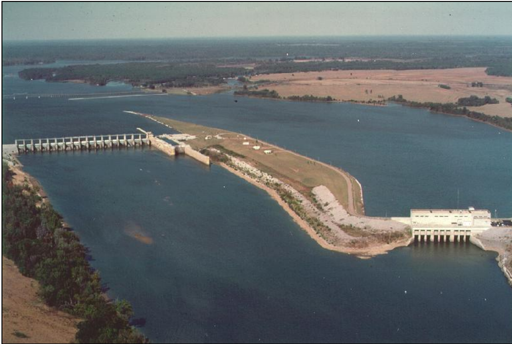
Figure 3. Millers Ferry Lock and Dam on the Alabama River. The lock measures 110 x 600 ft, and the powerhouse has an installed capacity of 75 MW.
