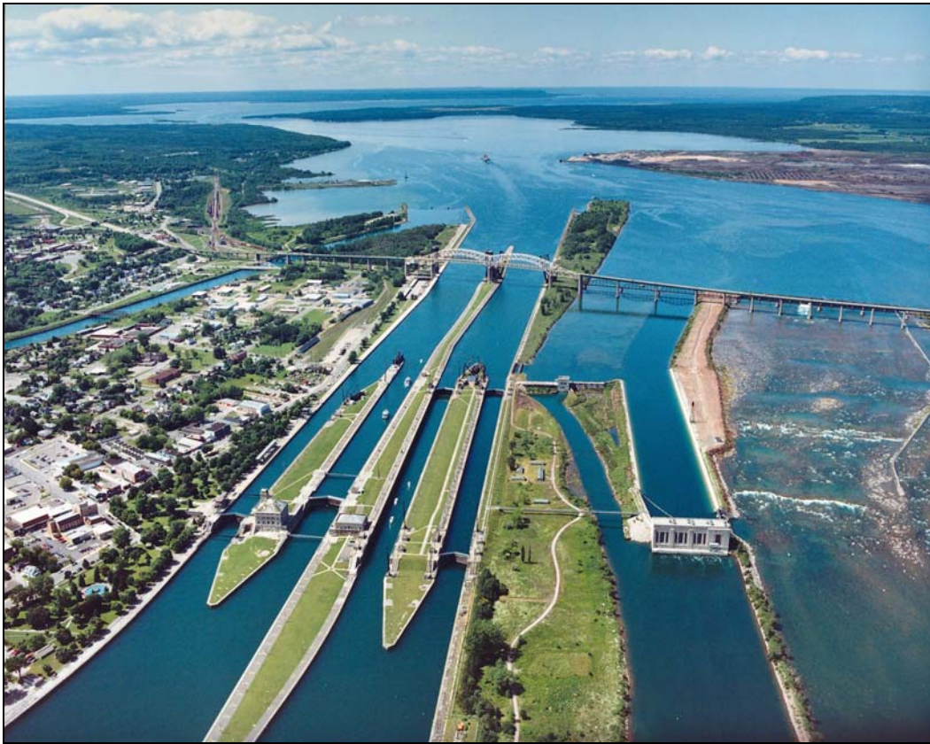
Figure 1. View of Soo Locks looking west towards Lake Superior. The lift is nominally 21 ft. Commercial freighters use the two left-most locks, respectively the Macarthur Lock (80 × 800 ft) and the Poe Lock (110 × 1200 ft). The third lock from the left (60 × 800 ft) is used mainly for summer pleasure craft, and the fourth is unused. The powerhouse has a 21-MW installed capacity, and the compensation works (upper right) controls the pool elevation.
