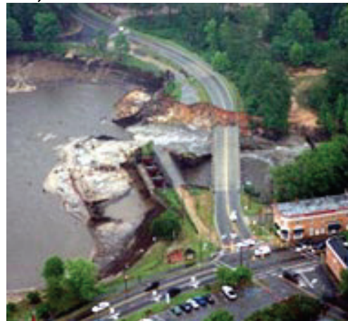
Figure 5. Rockfish Creek Dam failure, NC, 2003
