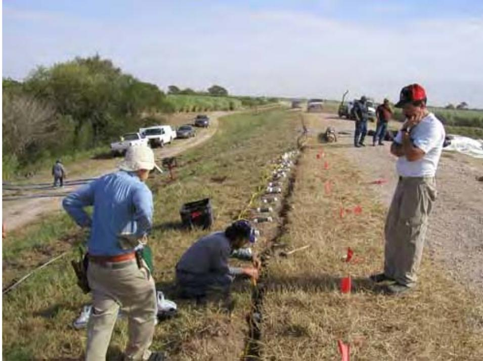
Figure 25. Installation of SP line (line A) along landside crest of levee. See Figure 15 for location of line A
