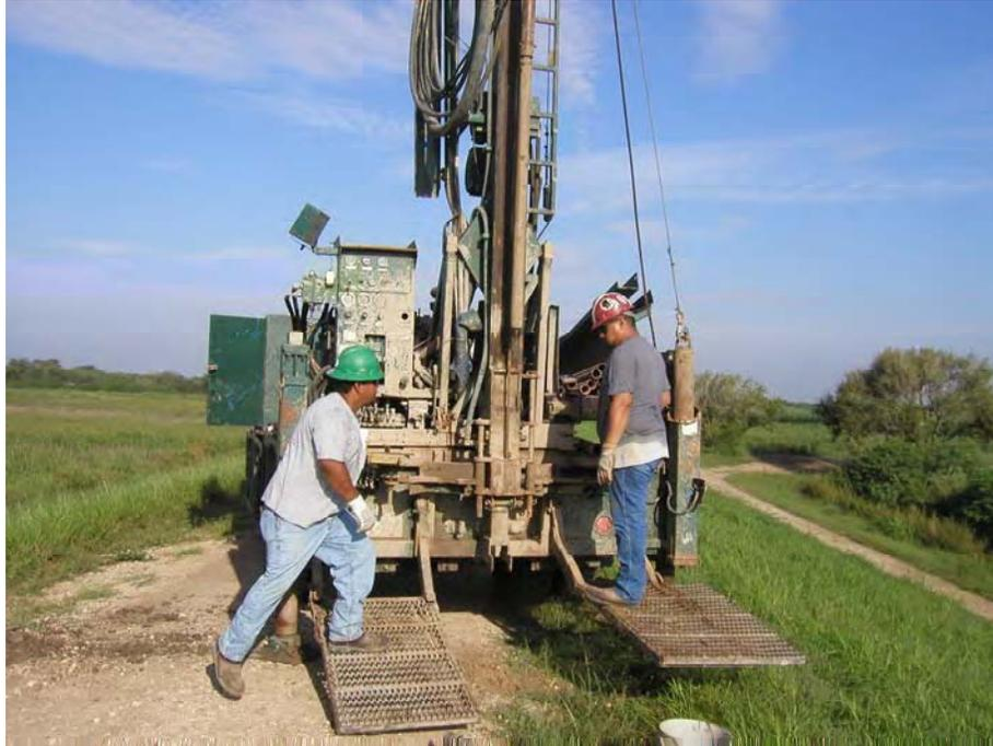
Figure 1. Soil sampling of levee at location SJ-TX-02. Boring SJ-TX-01 is located 10 ft to left on south levee crest.
