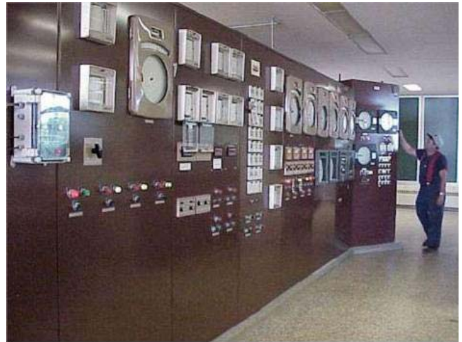
FIGURE 1. WATER PLANT CONTROL ROOM
