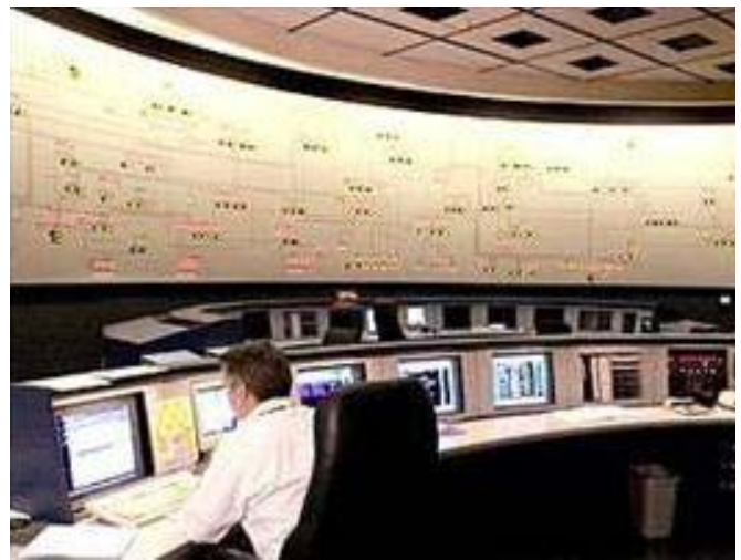
FIGURE 2. ELECTRIC POWER GRID CONTROL ROOM < http://msnbc.msn.com/id/3077316/ >
