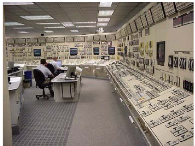
FIGURE 4. TYPICAL NUCLEAR POWER PLANT CONTROL ROOM < http://people.howstuffworks.com/nuclear-power4.htm >
