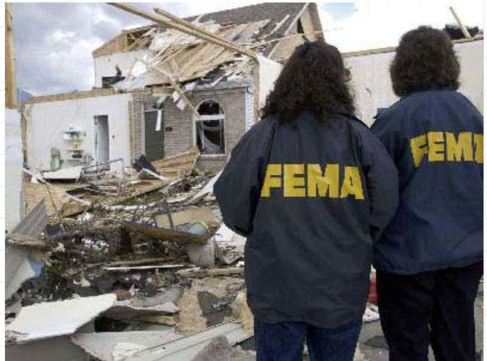
Photo Courtesy of FEMA [2]
