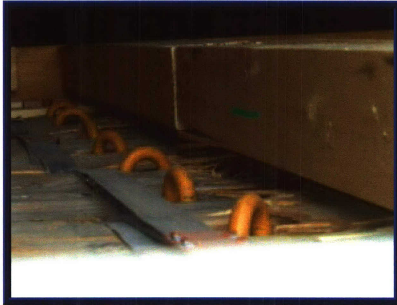
Photo 9. Damage to Top Board
