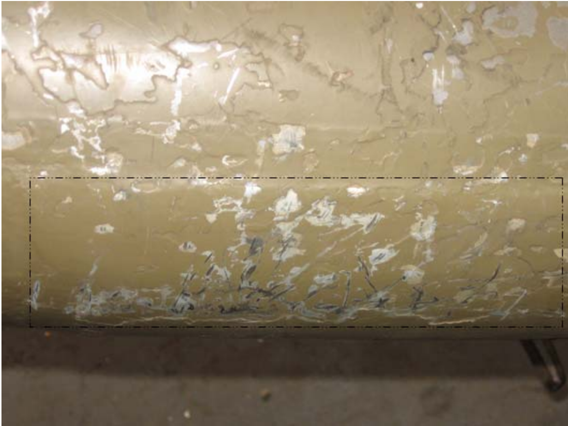
Figure 20 Reinforcement from region E, showing mechanical damage after three years of active service. No evidence was found of debonding in this or any of the other reinforcements
