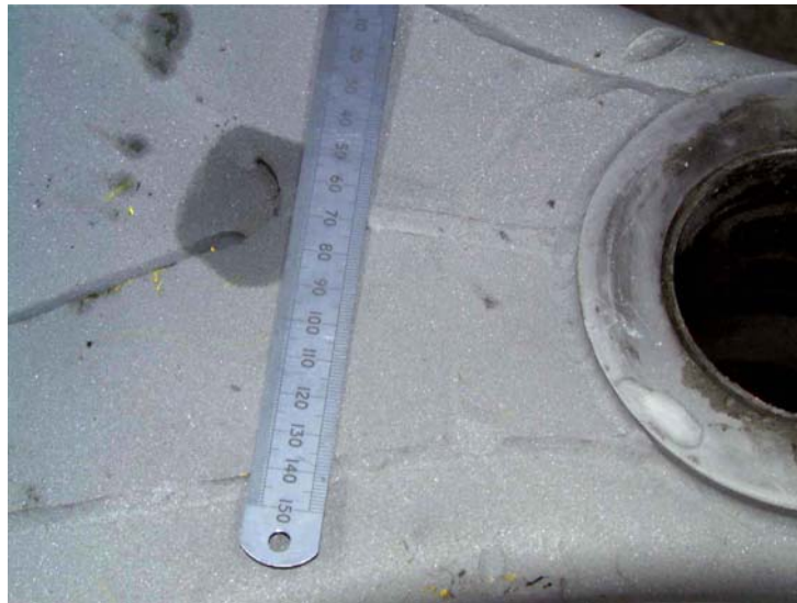
Figure 3 Gun trail showing chain scored region, selected for repair study
