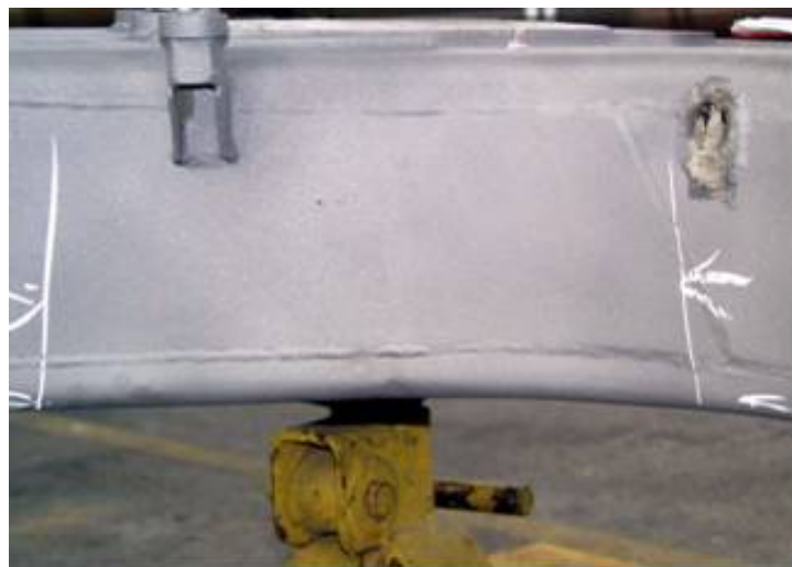
Figure 4 Gun trail showing damage to the base of the box section selected for repair study
