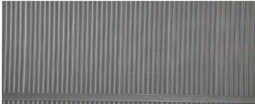
Figure 12: A photo of the atrium roof.
