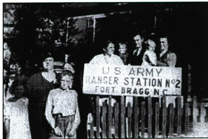
Figure 5. Ranger Station 2, 1937, Courtesy of Myra Mott Hanni
