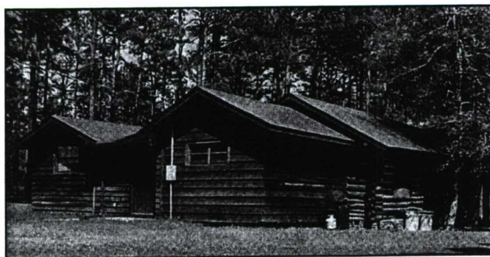
Figure 22. Ranger Station 5 at Camp Mackall, Photo by Lowell Stevens
