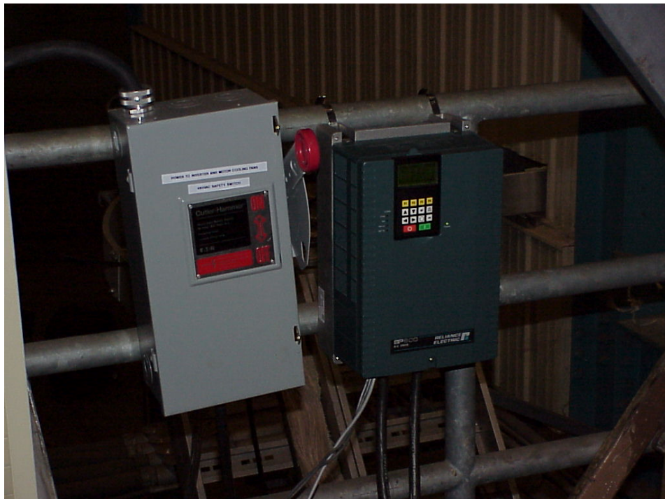
Figure 13. Reliance SP600 motor controller and power junction box
