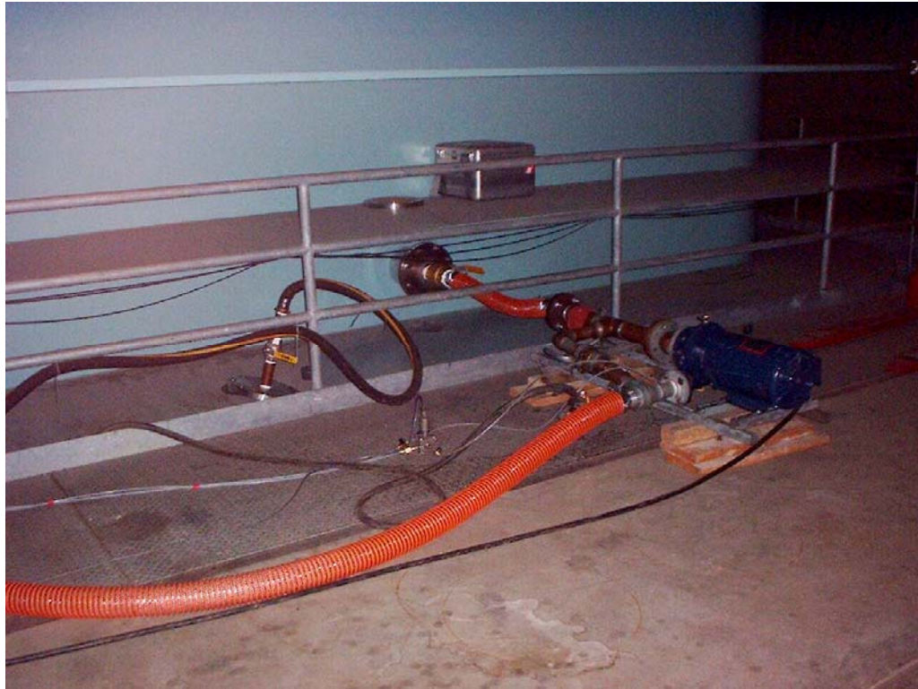
Figure 14. Inlet to the pump (Elbow#4) LCC Upstream Vertical Leg
