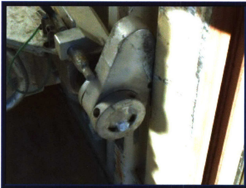
Photo 4. Cam not fully engaging shoring slot.
