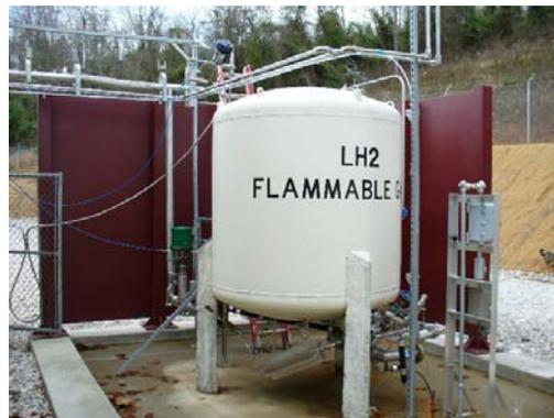
Figure 6: LH<sub>2</sub> tank
