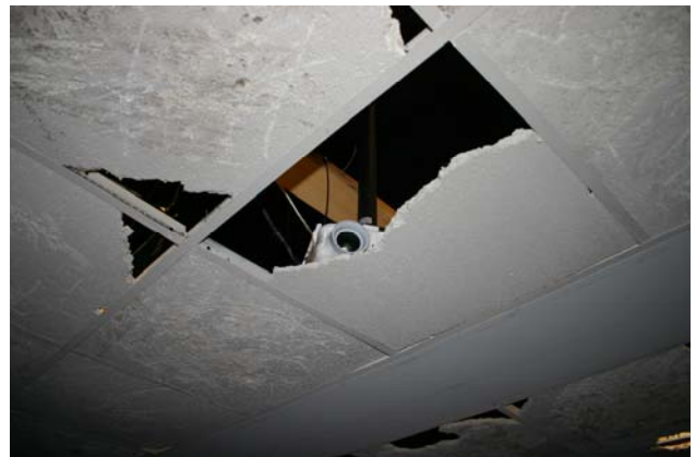
Fig. 2: Projector placed above the ceiling.
