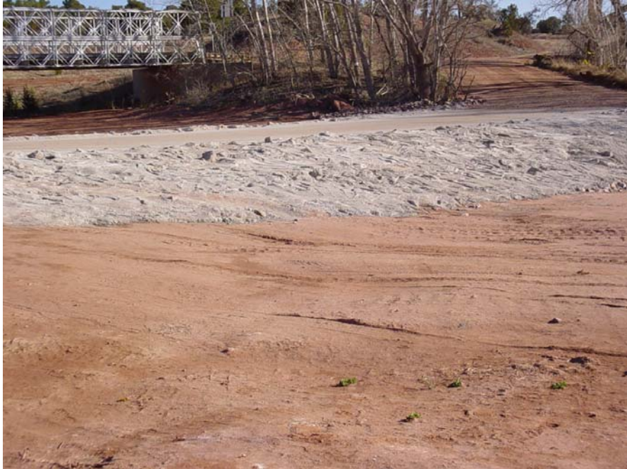
Fort Carson Low Water Crossing
