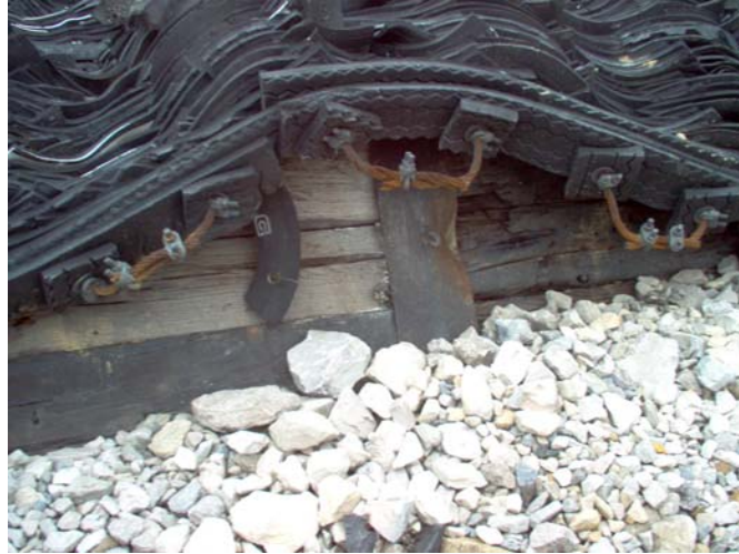
Wood and mount damage on battle position Cedar Creek MPTR at Fort Knox
