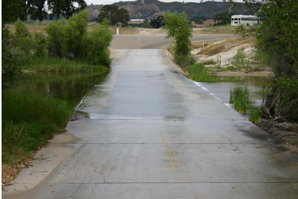
Fort Hunter Liggett Low Water Crossing
