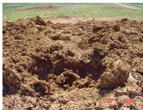
Ft Knox St Vith MPTR Projectile Impact Damage on SAT Berm
