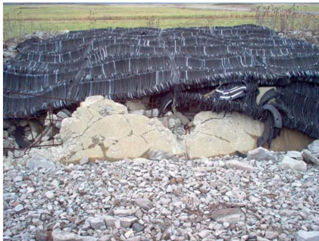
Concrete damage on battle position Yano MPRC at Fort Knox
