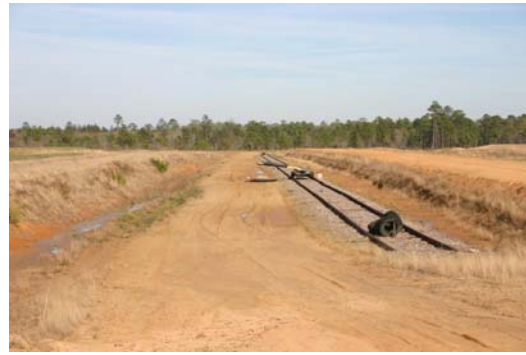
Ft Stewart Redcloud MPRC In Ground Remote Controlled MAT
