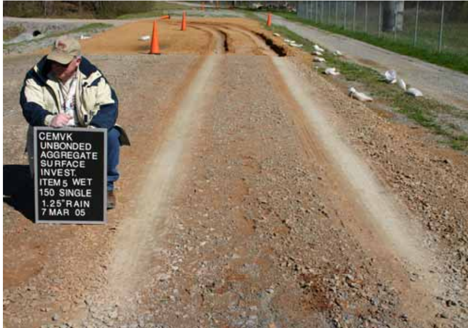
Photo C59. Item 5 (SSB), wet lane, maintenance test section, 150 passes with pickup truck
