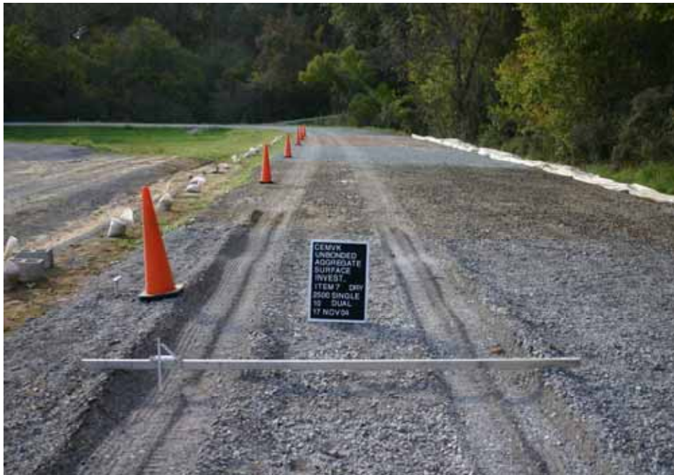
Photo C92. Item 7 (LST), dry lane, new construction test section, 10 passes with dump truck
