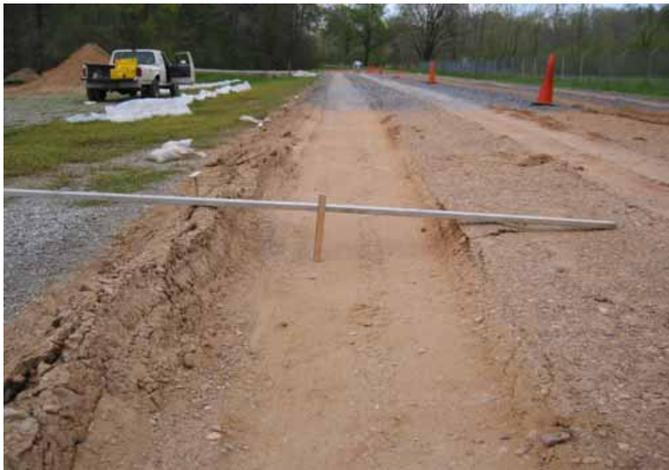
Photo C22. Item 1 (SCG), dry lane, maintenance test section, 200 passes with emulsion truck
