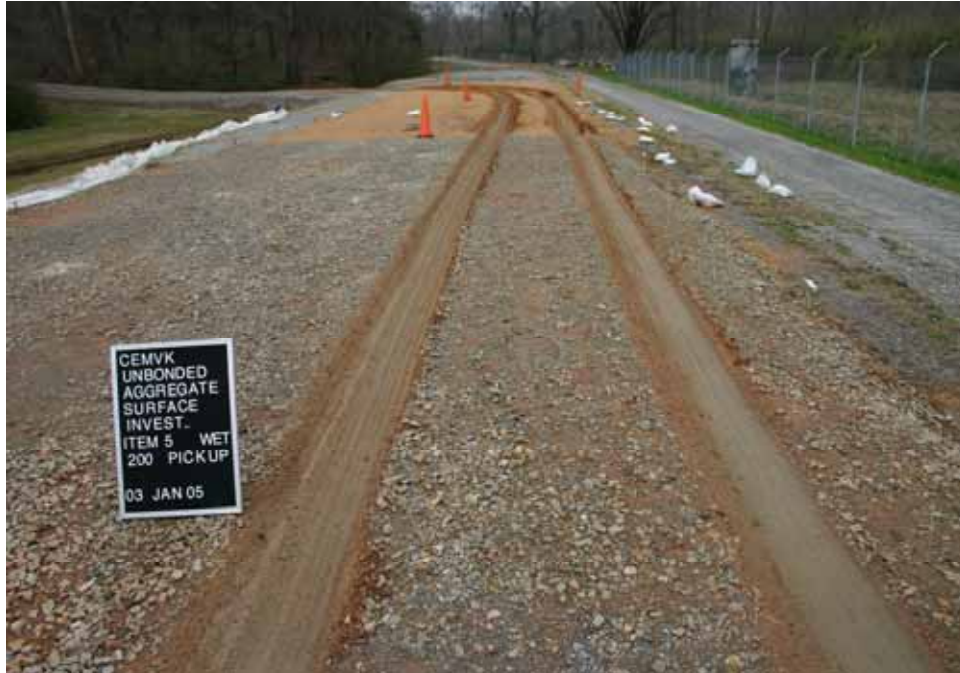
Photo C39. Item 5 (SSB), wet lane, maintenance test section, 200 passes with pickup truck
