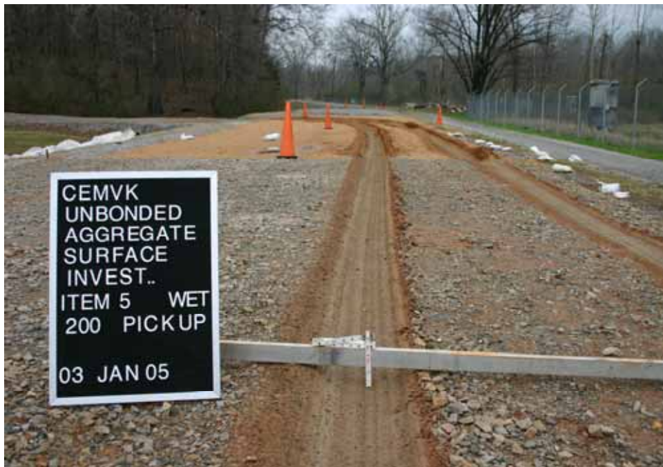
Photo C40. Item 5 (SSB), wet lane, maintenance test section, 200 passes with pickup truck
