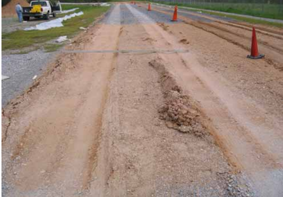
Photo C21. Item 1 (SCG), dry lane, maintenance test section, 200 passes with emulsion truck
