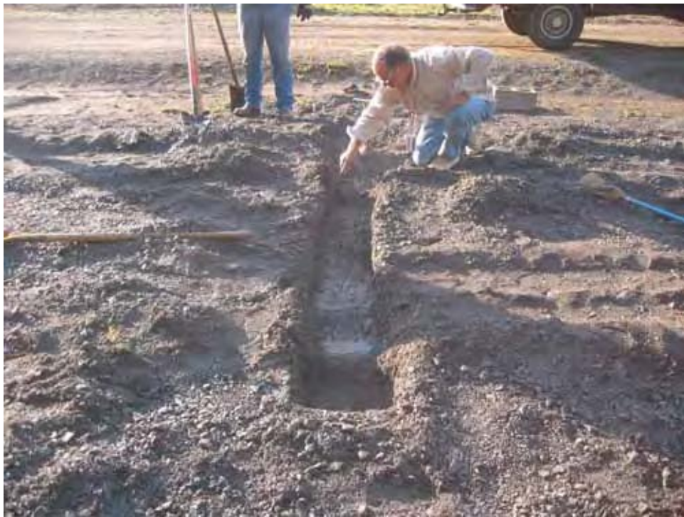
Photo 4. Wet subgrade under Item 7 (LST) surface aggregate
