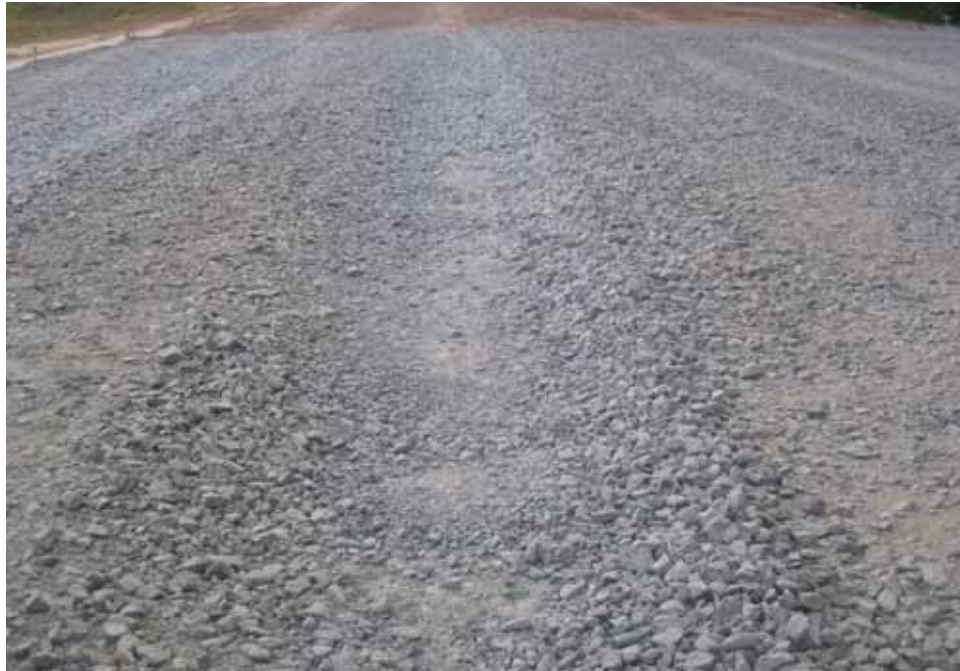
Photo C78. Item 9 (IGN), dry lane, new construction test section, 500 passes with pickup truck
