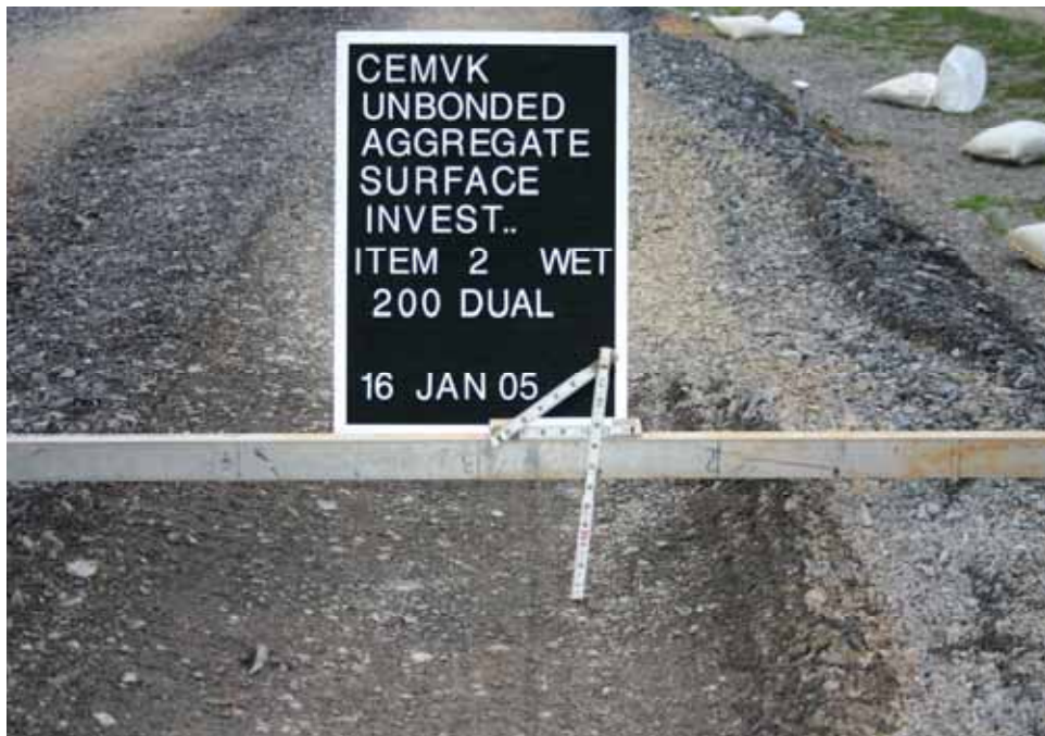
Photo C44. Item 2 (LST), wet lane, maintenance test section, 200 passes with dump truck
