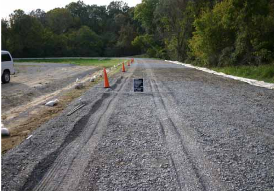
Photo C93. Item 7 (LST), dry lane, new construction test section, 10 passes with dump truck
