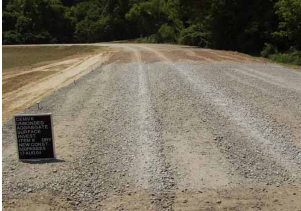
Photo C77. Item 9 (IGN), dry lane, new construction test section, 500 passes with pickup truck
