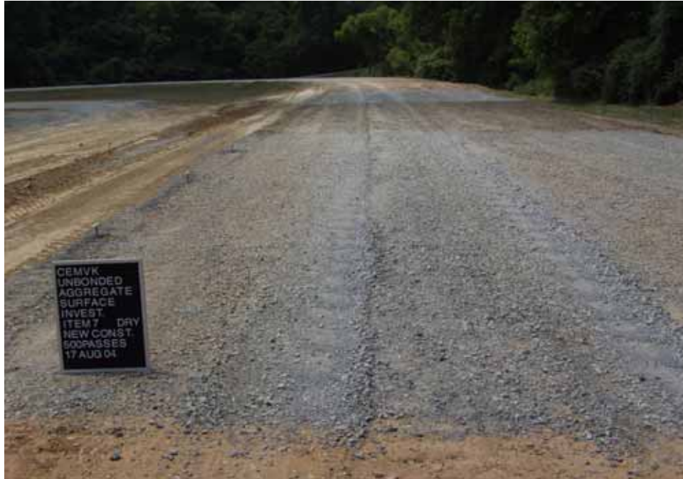
Photo C73. Item 7 (LST), dry lane, new construction test section, 500 passes with pickup truck
