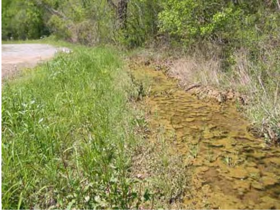
Photo 3. Ponding of water along outside shoulder
