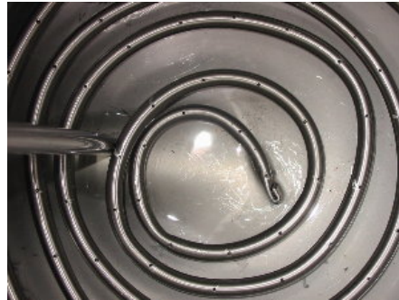
Fig. 1. Top view of sparge spiral in the bottom of the fuel preparation tank.
