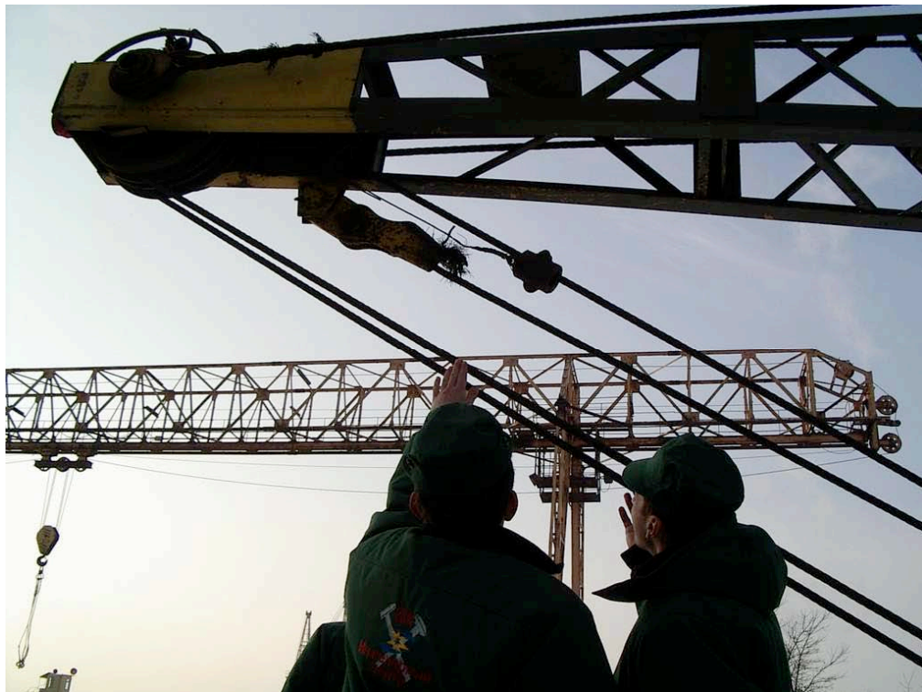
Figure 5.10d: Crane Examination Techniques – Horizontal Examination.
