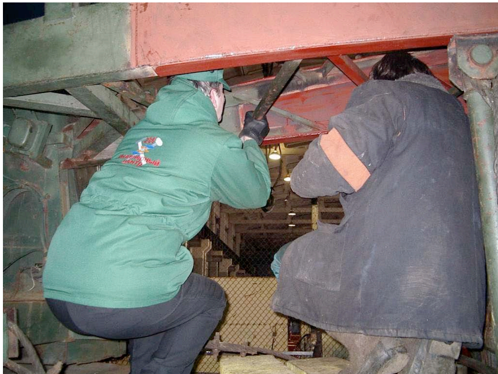
Figure 5.9b: Crane Examination Techniques – Fabrication Methods. The fabrication specialist is shown (right) working with the MOD student (left) to identify the methods used to repair the structure.
