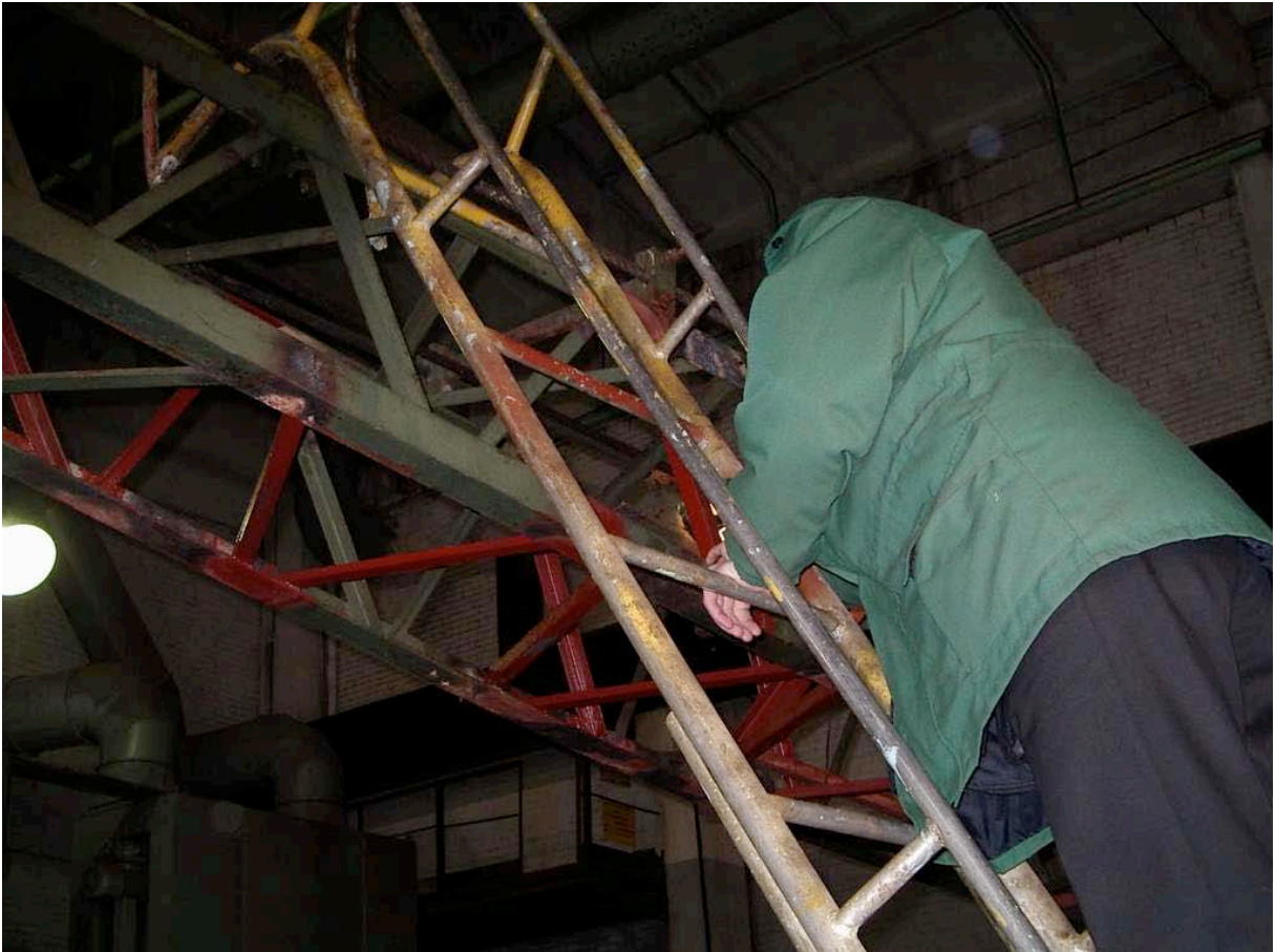
Figure 5.7: Crane Examination Techniques. In this figure, the MOD student is moving along a truss section examining the surface conditions for individual welded sections. The student is also applying capillary methods to chemically amplify the surface deformation. In this manner, the principal cracks and surface deformations may be identified and marked for secondary examination using the surface hardness testing instruments and the ultrasonic defectoscopes.
