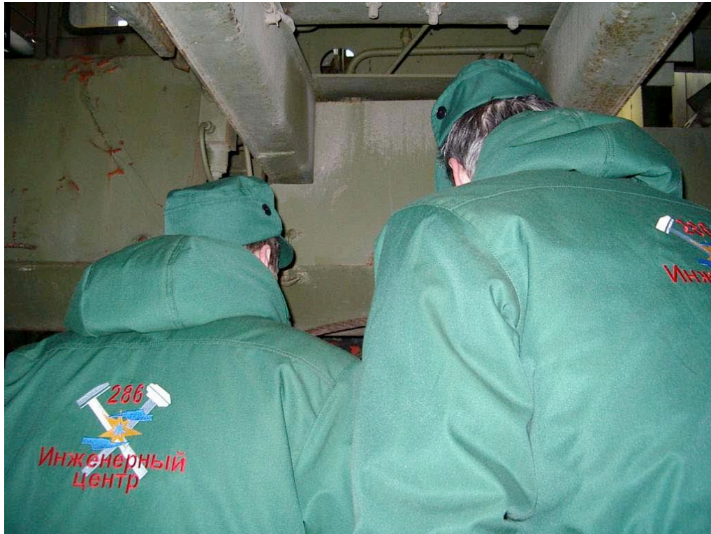
Figure 5.6a: Crane and Hoist Service Life Determination.
