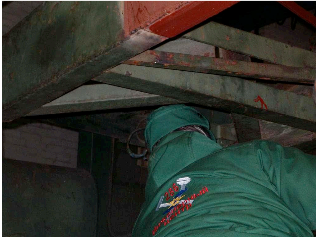
Figure 5.9a: Crane Examination Techniques – Undercarriage Examination.
