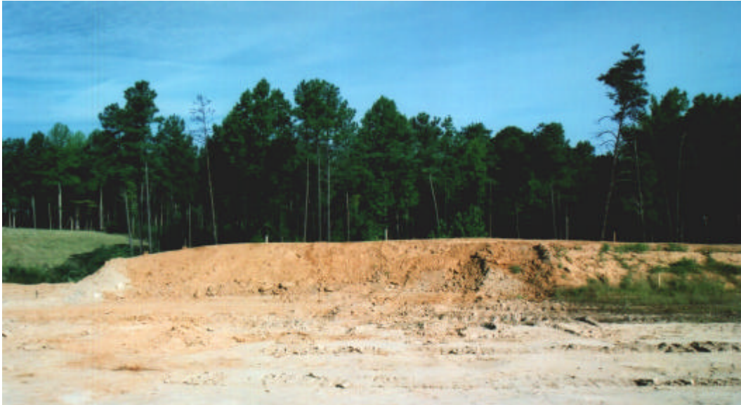
Figure 8. Berm at Test Site 2
