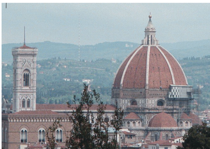
Fig. 1 Built from the bottom up, a single brick at a time. (a) The Great Wall of China, started in 700 BC, is 5600 km in length and each brick is \sim 10 \times 20 \times 30 cm; (b) Florence's 14 th century Duomo, many small bricks and tiles add up to a majestic dome \sim 44 m in diameter.
