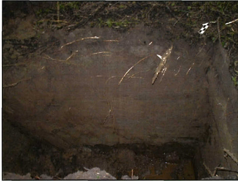
Figure 21. Photo of a typical backhoe trench excavated within the access road project item.
